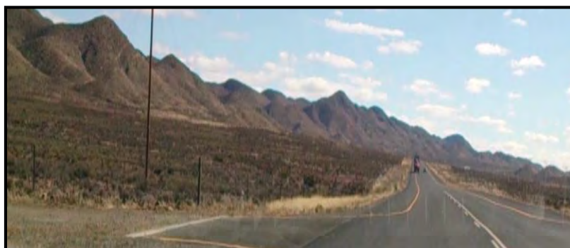
Figure 5.7: Absence of streetlighting on the N1 highway
