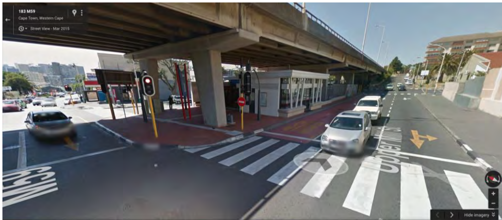
Figure 17: Google street view of Gardens MyCiTi station under M3 Expressway
