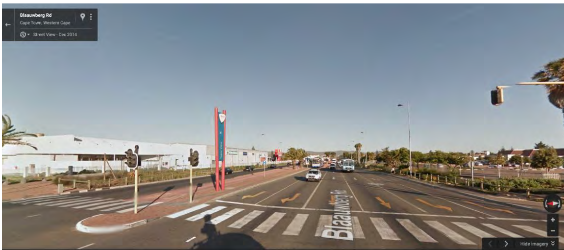
Figure 23: Google Street View of Table View MyCiTi station
