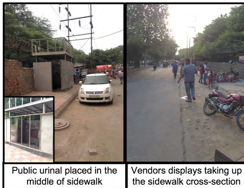
Figure 57: Sidewalk obstruction in Mandangir/Dakshin Puri
