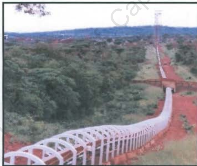
Figure 1.1: Zisco Overland Conveyor System
