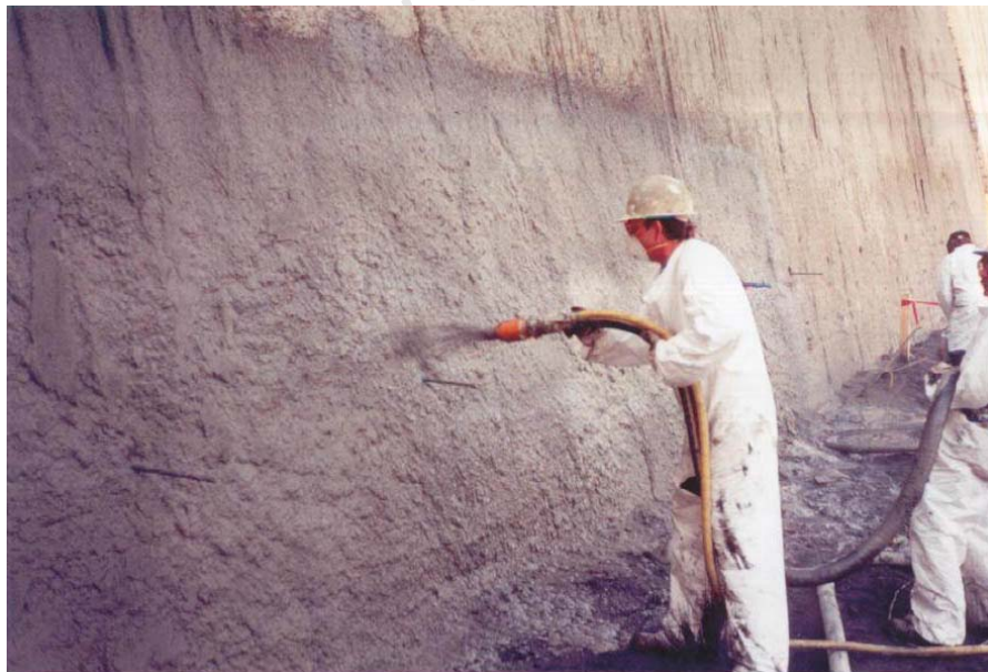
Fig. 2.2: Shotcrete applied on vertical wall www.mudjacking.com
