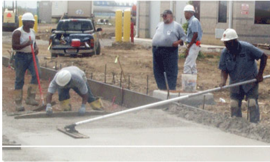
Fig. 2.1: Overlay application on slabs-on-grade www.munic.org
