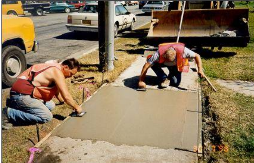
Fig. 2.3: Overlay repair on concrete footpath www.gaddis&sonnic.com
