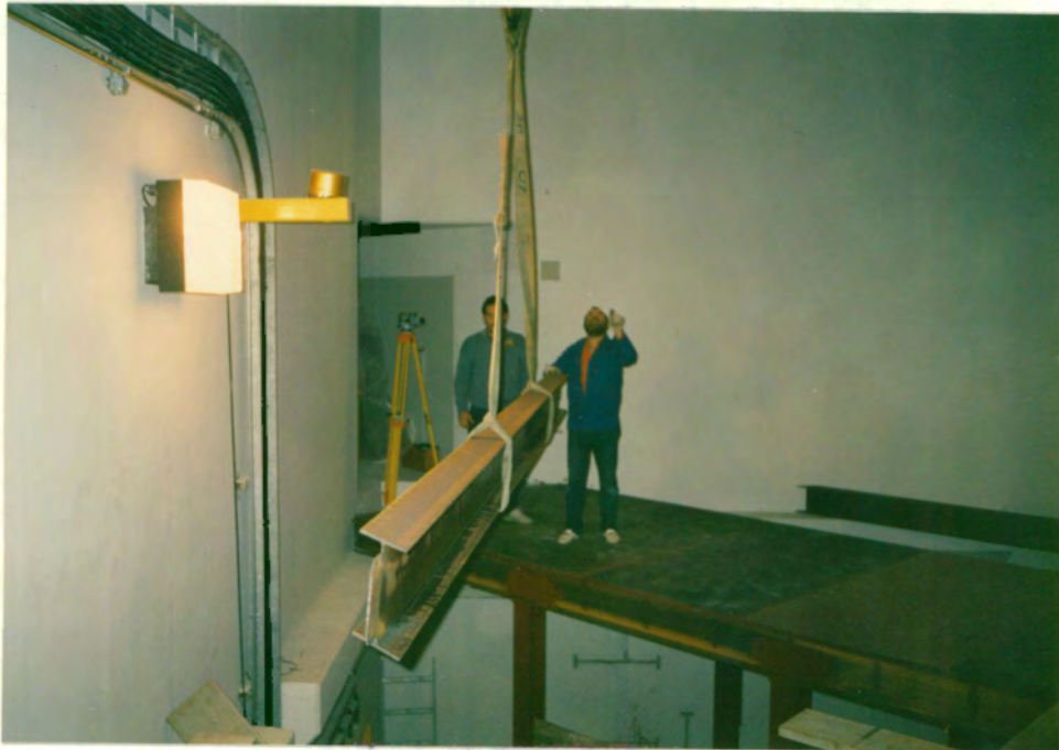
Figure 7.3. The raised floor under construction
