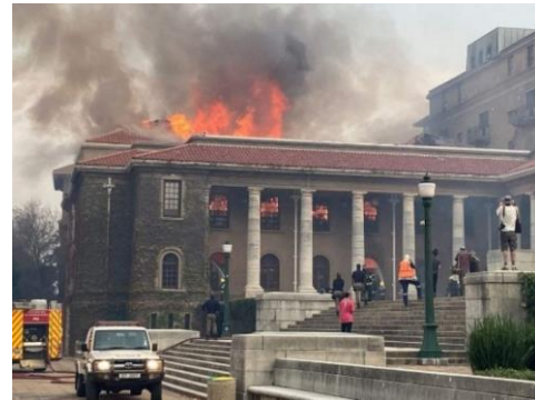
Figure 2: University of Cape Town, Jagger Library on fire (Charles, 2021).
