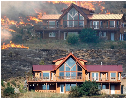
Figure 70: A home that is wildfire resistant, due to non-combustible materials used, steel gutters, sealed doors and windows, doors decks chimneys (Howell, 2020).
