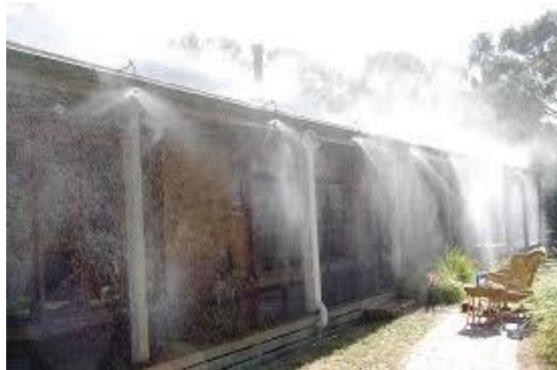
Figure 71: A home with a sprinkler system to stop burning embers (Terramatrix, 2020).
