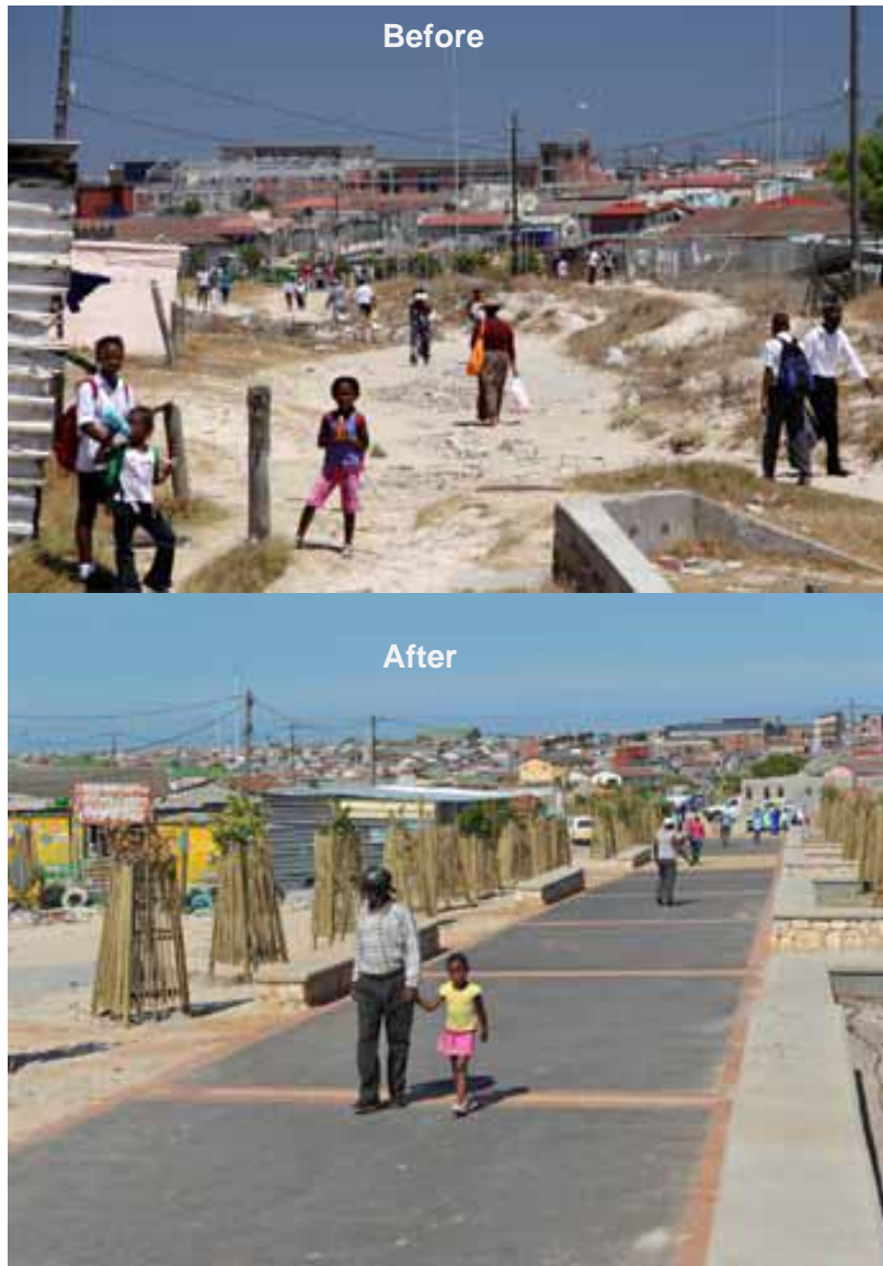
Figure 26: road or footpath, doubling as a fire break, after intervention (CoCT, 2014).
