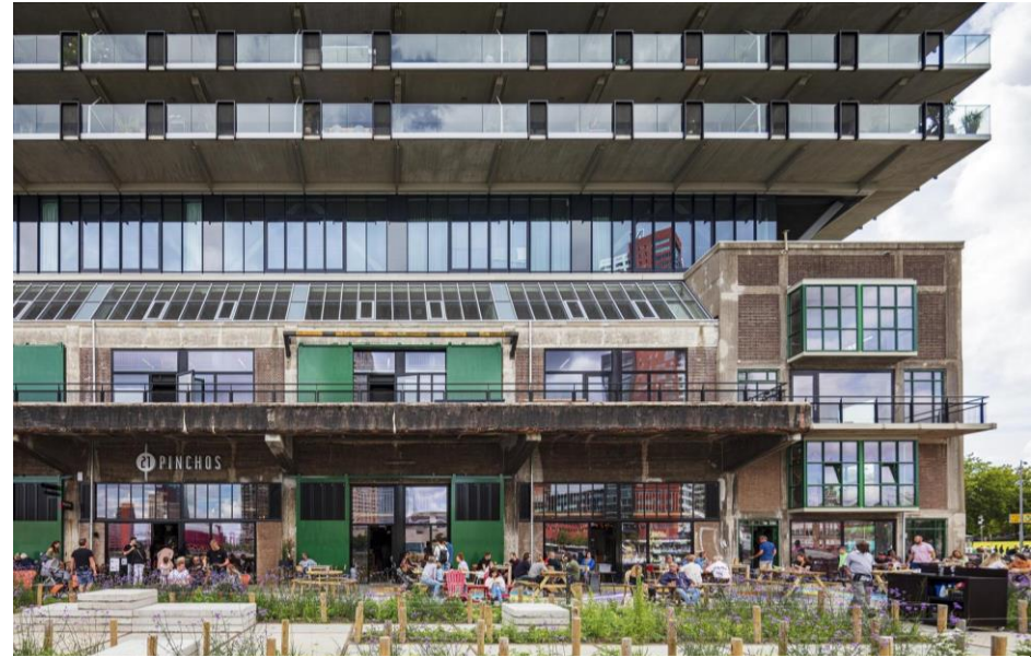
Figure 19 Fenix 1 as seen from the public edge, giving insight into the typical use of set space, in contrast with the more quiet and private upper part of the facility. (Marc Goodwin, 2020)
