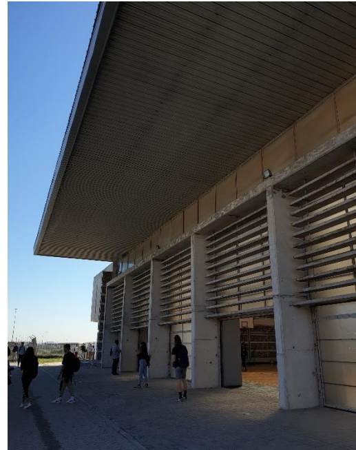
Figure 23 External view of the Thusong Service Centre, Standing outside the Central court and operable doors. (Ruben van Biljon, 2019)
