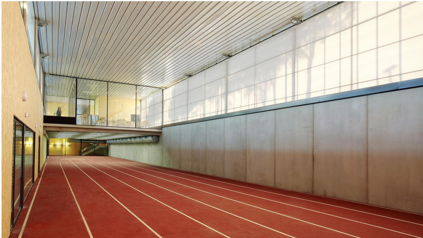
Figure 7 Basement level of the Calvia Running track in Spain. This image gives a good understanding of the conditions of the indoor spaces. This section forms part of a warmup track for athletes. (Jose Hevia 2010)
