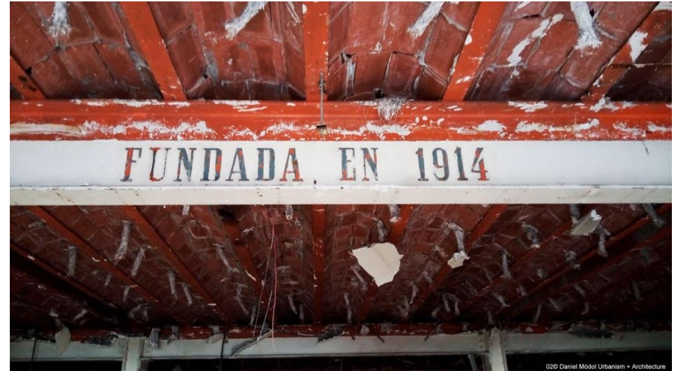
Figure 30 Image of the Original steelworks present on site of LOOM Coworking space that had been restored to become the green steelworks. (Daniel Modol, 2022)
