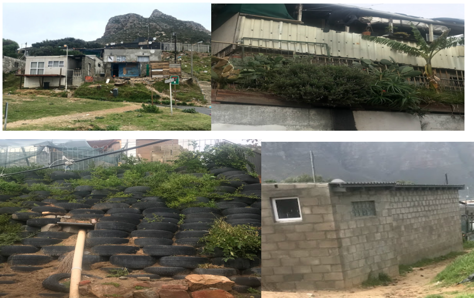
Figure 4: Different building structures in Hangberg designed to deal with flooding in the informal settlement. Source – Fieldwork pictures.
