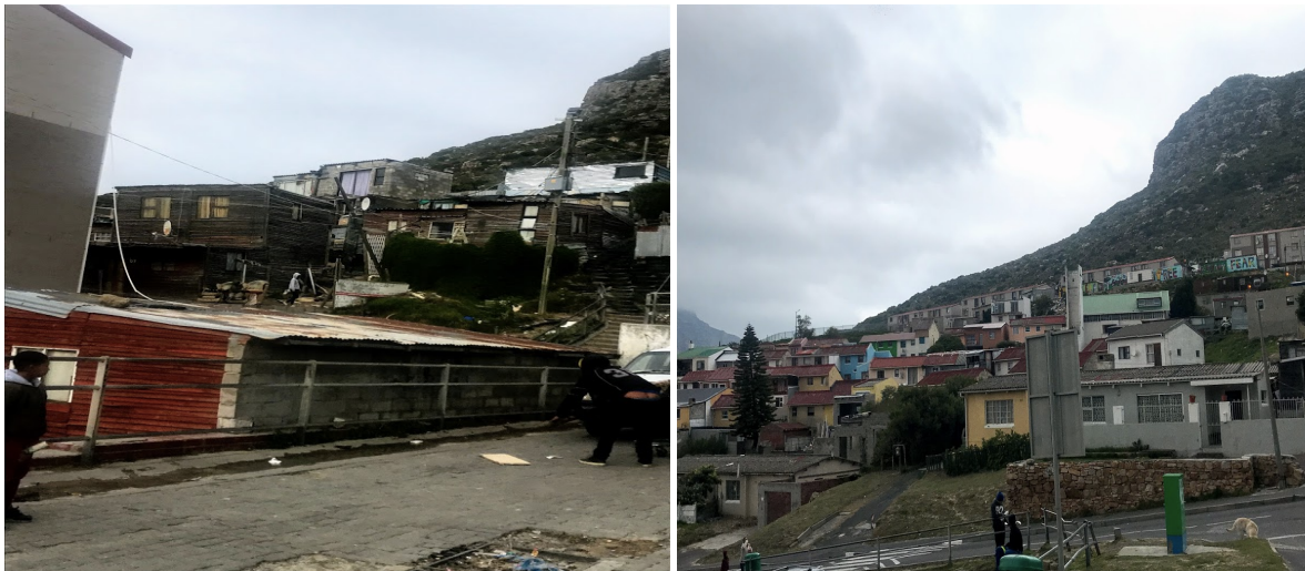
Figure 11: Different structures in Hangberg: Left structures built by residents in the informal area to meet their needs, Right structures constructed by the City of Cape Town. Source – Fieldwork pictures.
