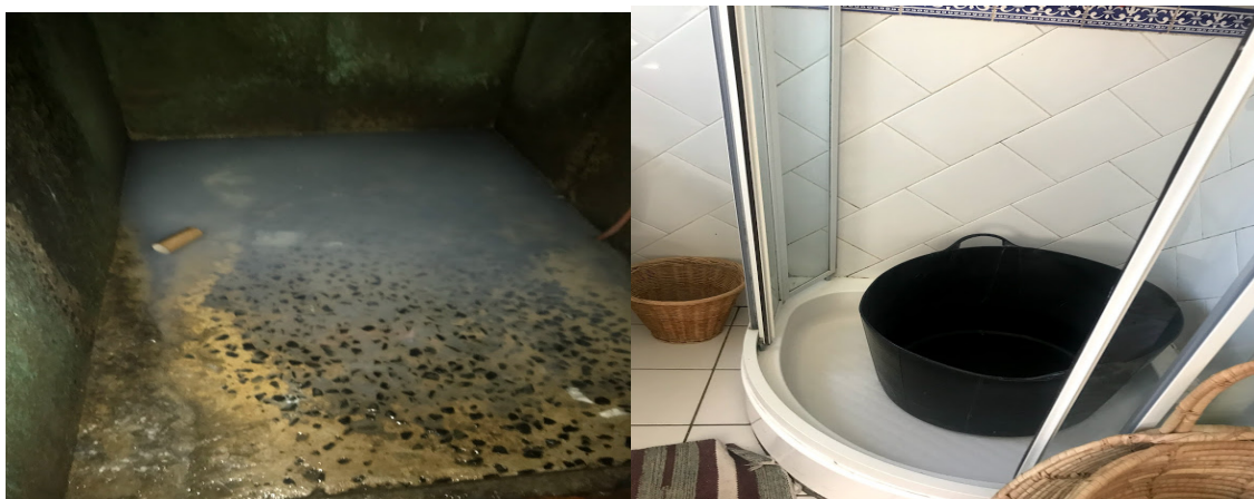
Figure 5: Picture showing sanitation facilities. Left - shared shower area in Imizamo Yethu; right – private shower area in Bokkemanskoolf Estate. Source- fieldwork pictures.
