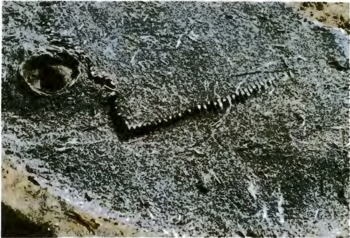
Figure 5.1.4 (a). Photograph showing the plane of fracture through reinforcement.
