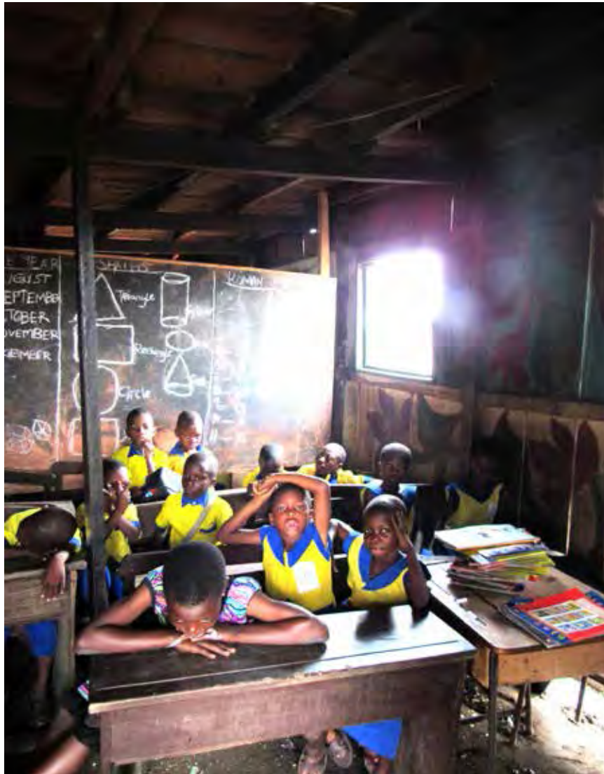
fig. 57 The dilapidated Makoko Whyinna Primary School.
