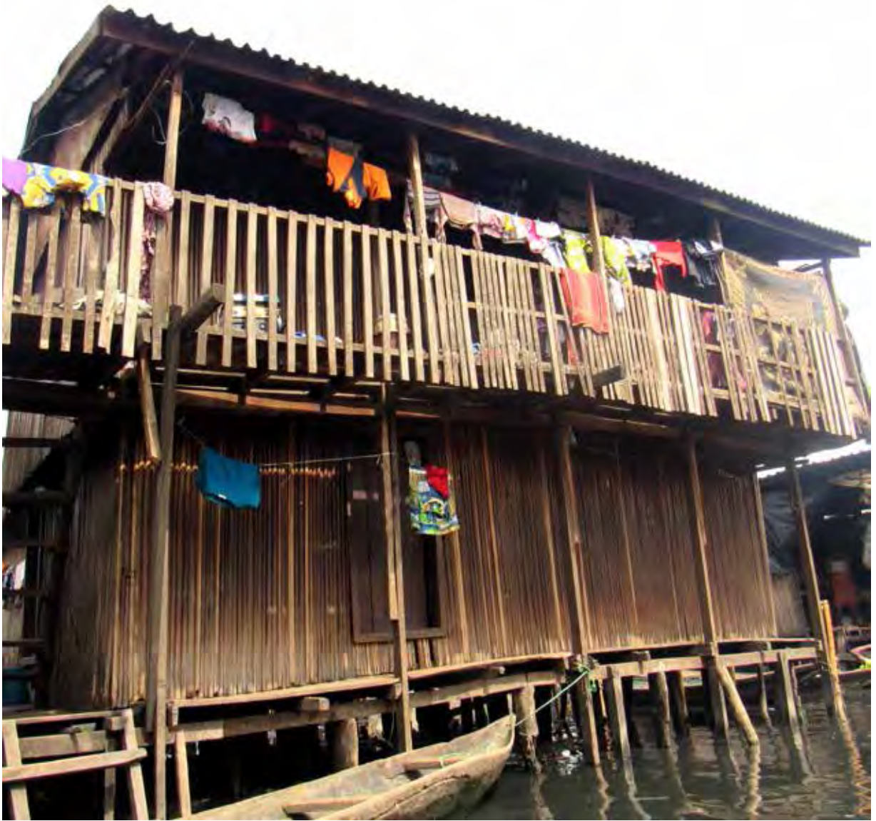
fig. 47 A unique double-storey dwelling in Makoko. On observation most are single-storey.
