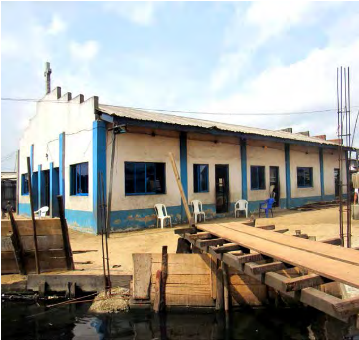
fig. 54 A church beside the canoe hiring point. Most of the churches in Makoko are built with concrete blocks contrasting the timber used in building most Makoko structures. The churches define public space.
