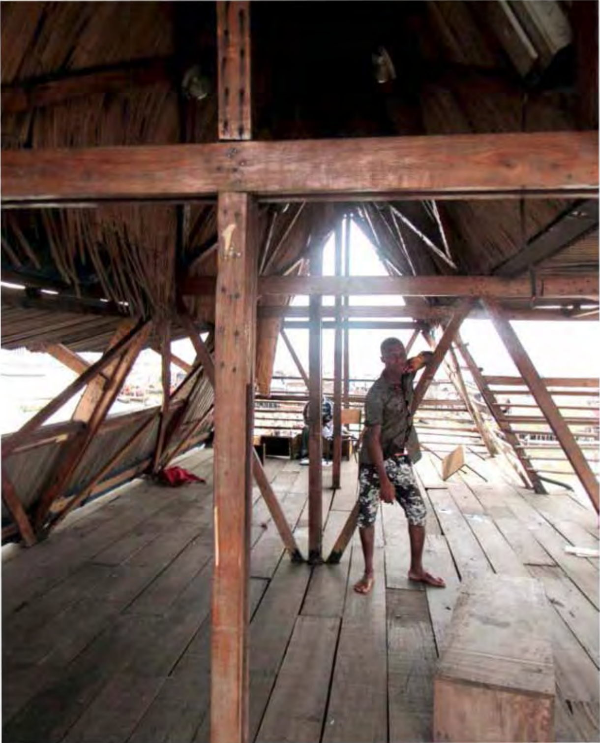
fig. 61 Timber structure of the Floating School. A unique detail in Makoko.
