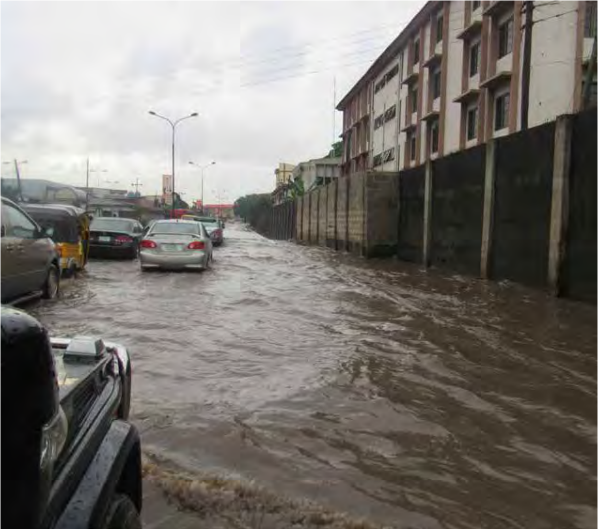
fig. 17 Flooding on Herbert Macaulay Way. A road close to the Makoko precinct.
