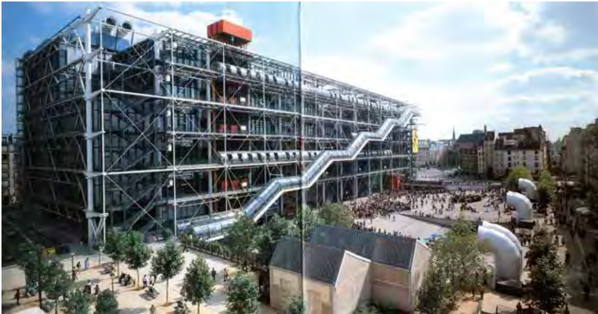
fig. 74 The externalized cascading staircase of the Pompidou centre allows for efficient movement between levels.
