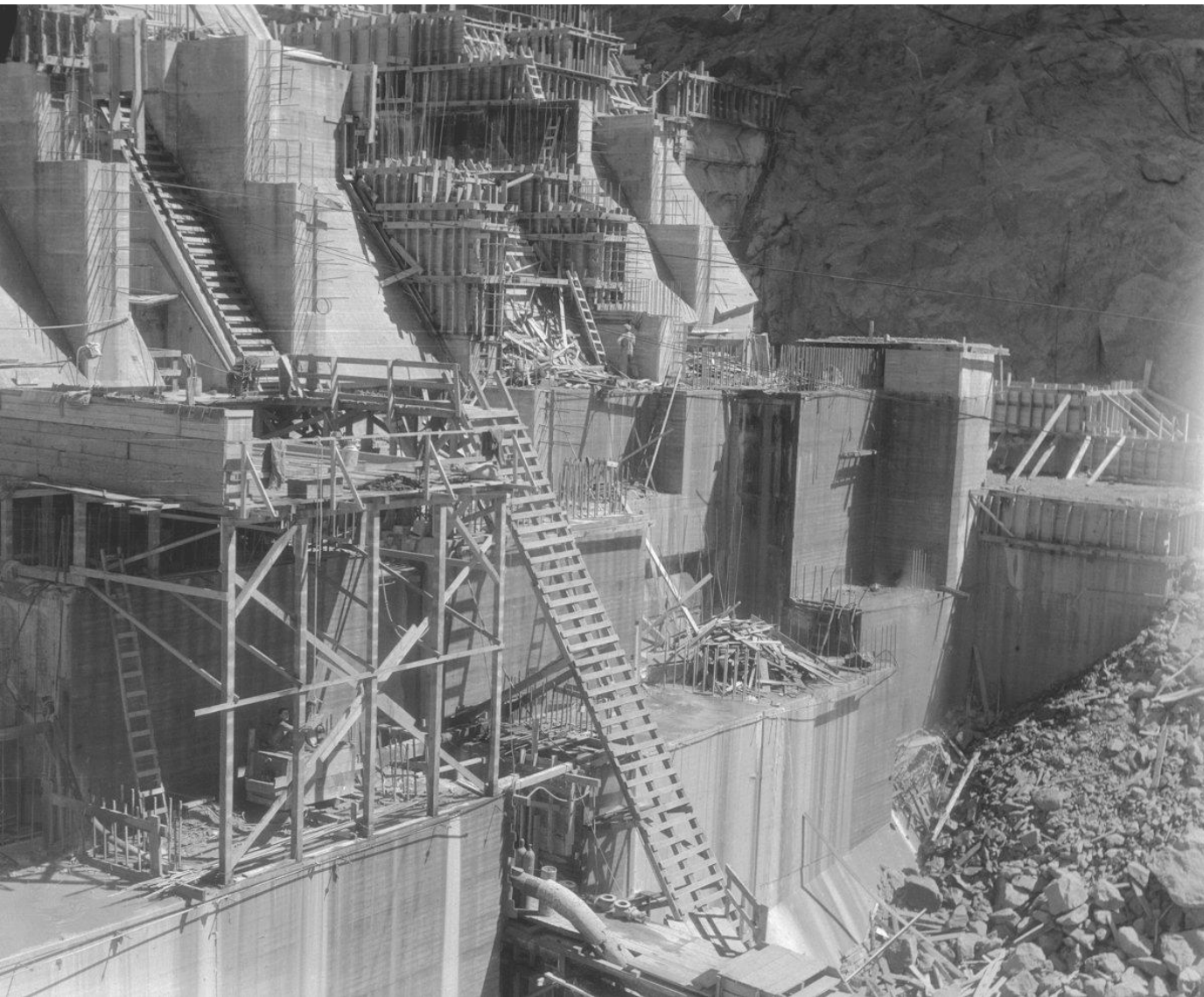
39. Scaffolding during dam construction.
