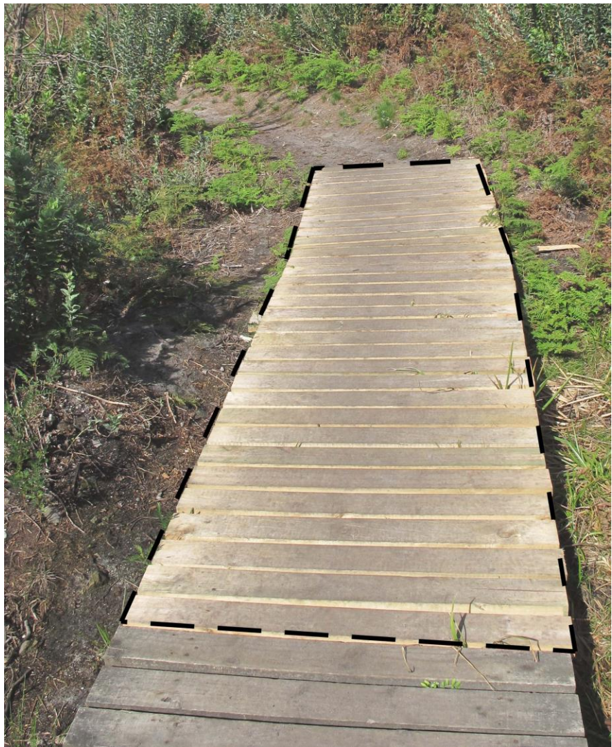
16. Reconstructed River Trail.
