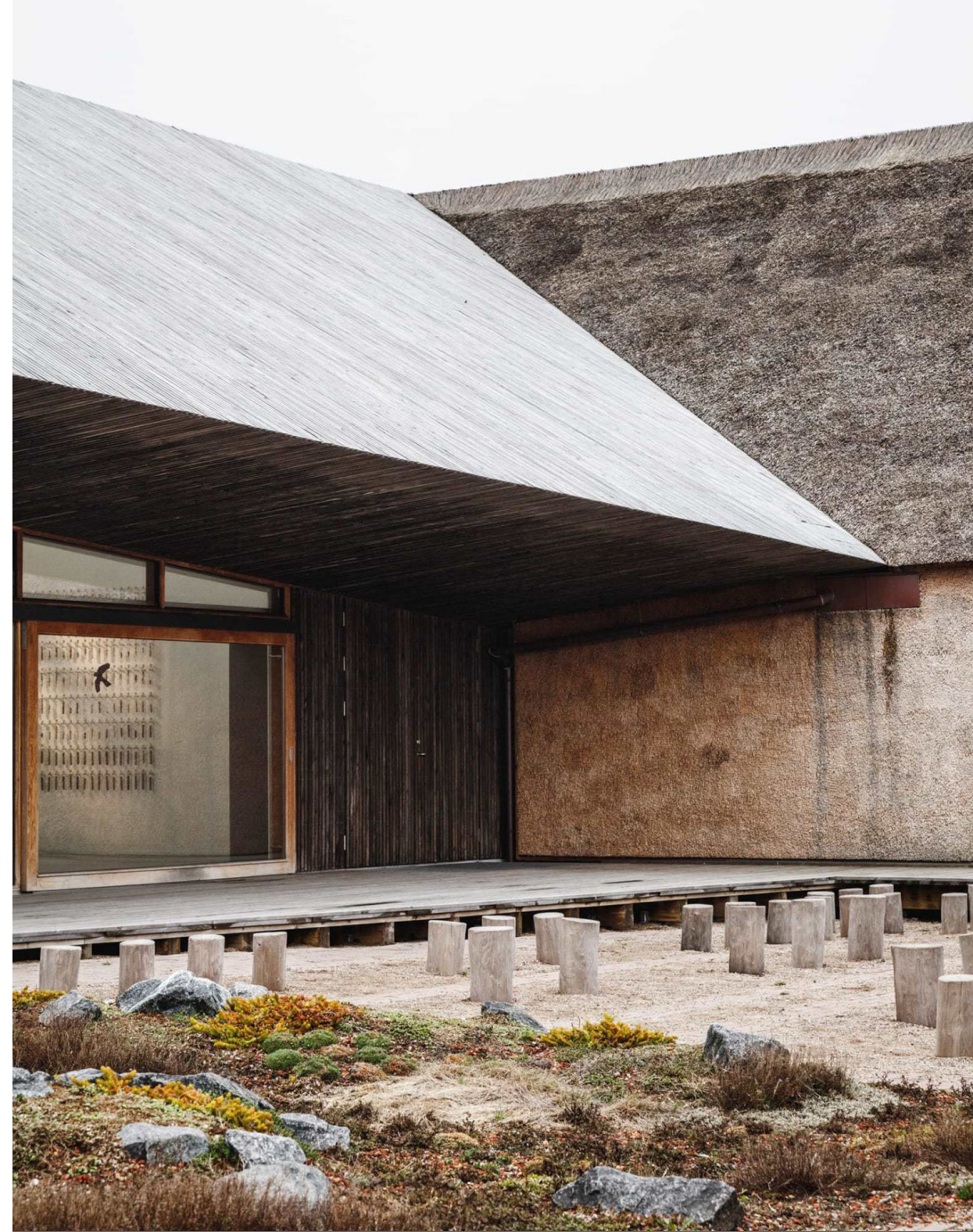
Figure 5.2.1: Courtyard exhibition with a view towards an interior exhibition. (Source: Rasmus Hjortshøj, 2017)
