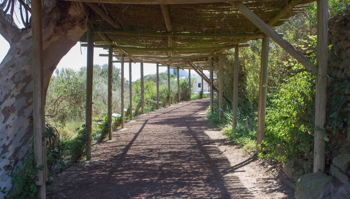
Figure 5.1.4: Covered entrance walkway leading to arrival courtyard. Source: author.
