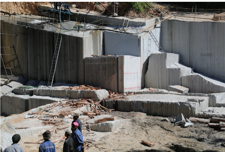
Fig. 31. Photographs of the De Hoop Quarry, Paarl
