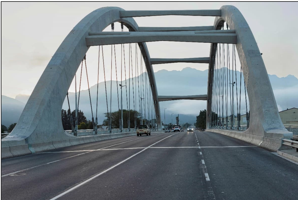
Figure 3-8: Western Side view of cables on the arch ribs. Photographed by Terry February for AECOM SA, 2022
