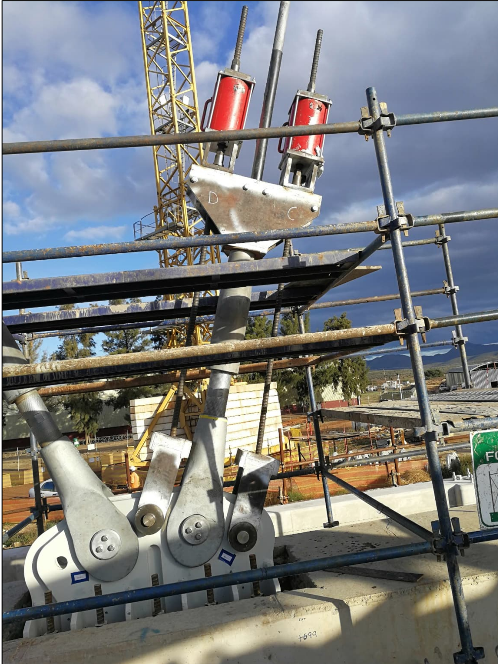
Figure 4-4: Pair of hydraulic jacks (in red) used to tension a cable
