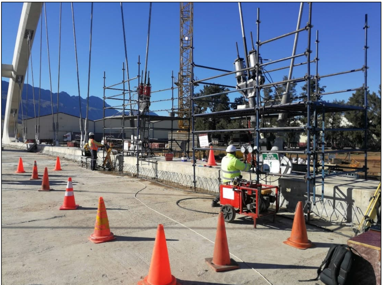
Figure 3-9: Tensioning of cable S12 and S13 pair
