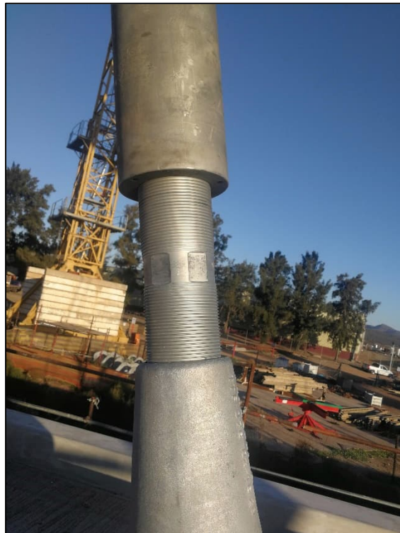
Figure 3-13: Threaded turnbuckle region adjusted during tensioning
