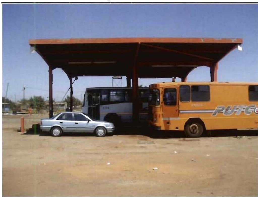
Photo 8.12 View of USTs from 10m looking south
