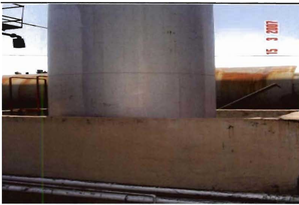
Photo 8.7 View of Shell 9,400 litres AST from 10m looking west
