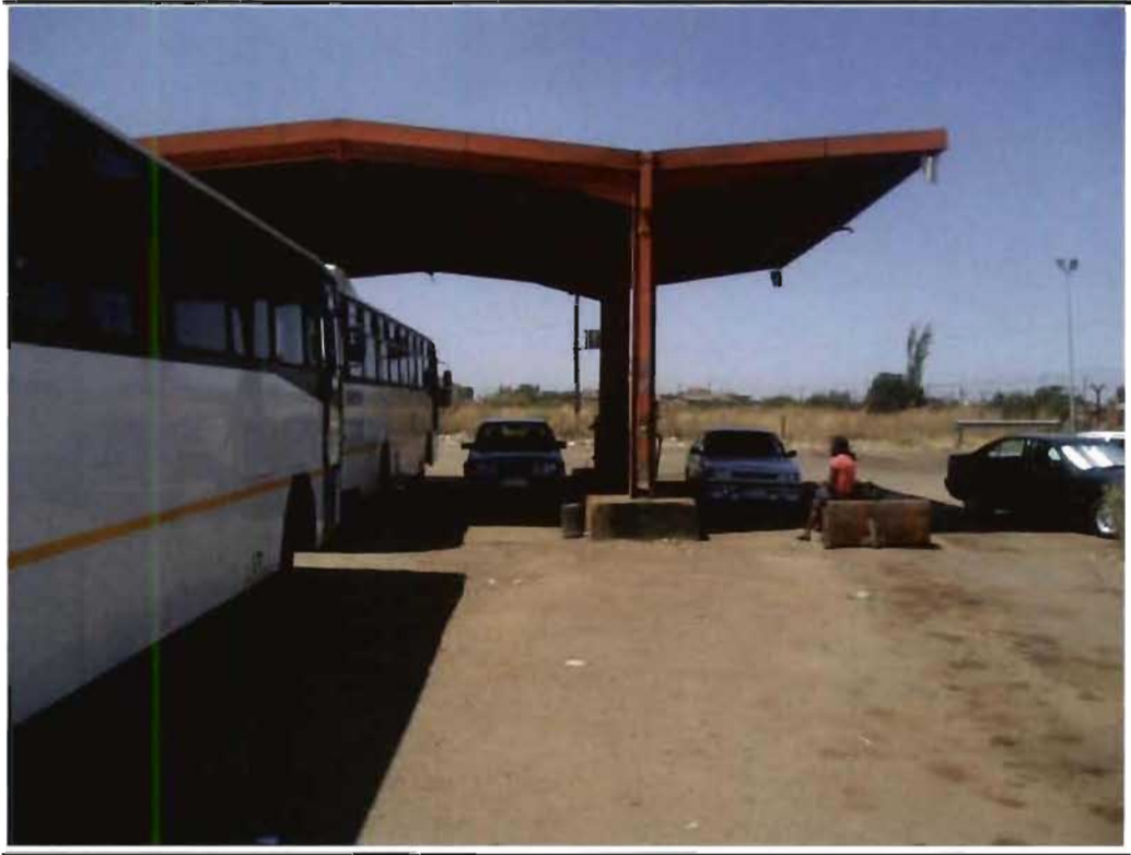
Photo 8.10 View of USTs from 10m looking east (1 of 2)
