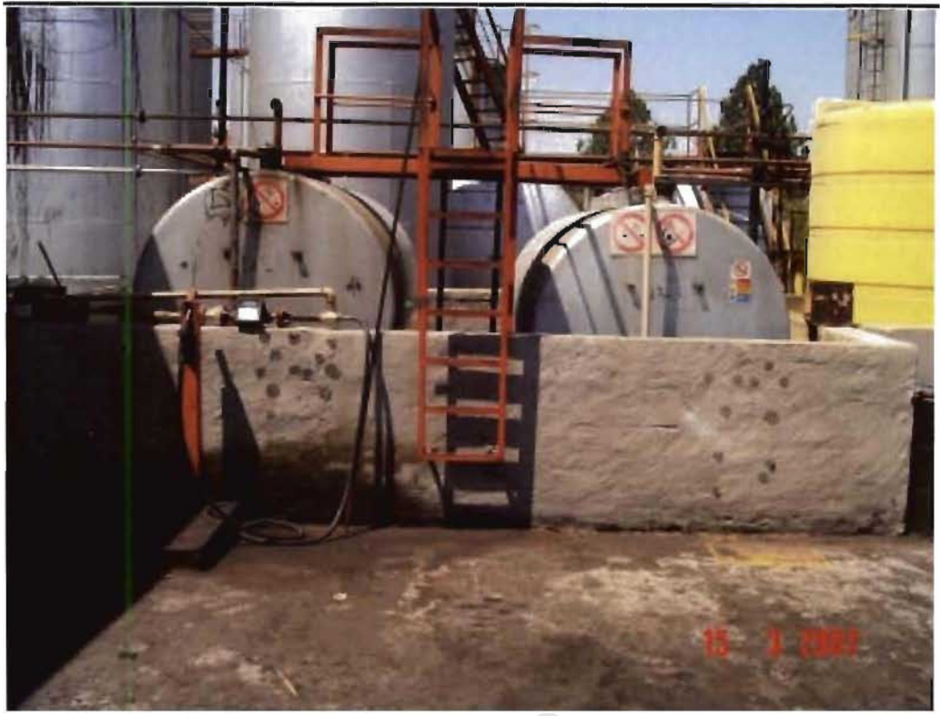
Photo 8.1 View of Shell-AST 2 x 9,000 Litres from 10m looking north
