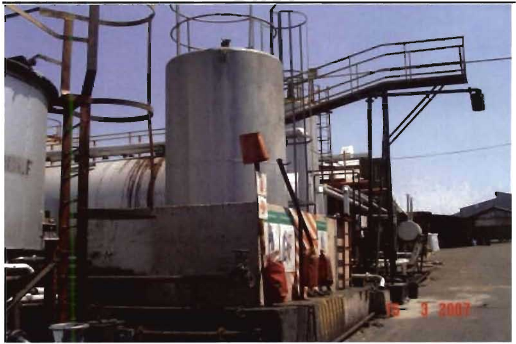
Photo 8.2 View of shell -9,4 00 litre AST from 20m looking north
