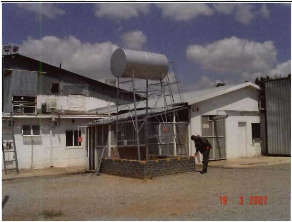
Photo 8.2 Site 1 - view of the tank from 50m looking north east
