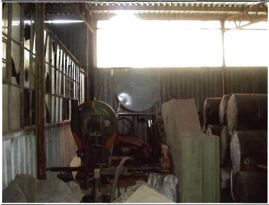
Photo 8.1 View of the tank from 10m looking north
