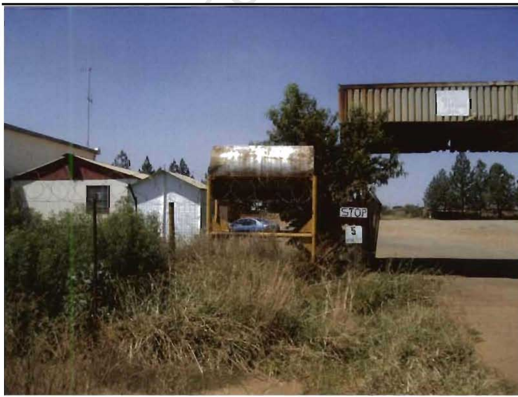
Photo 8.6 View of AST (tank 2) from 10m looking east
