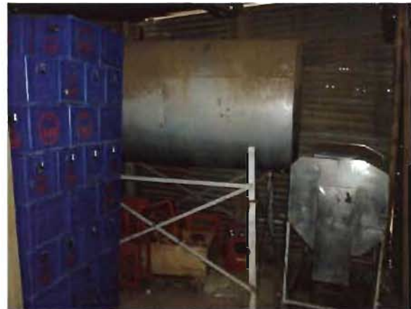
Fig 8: AST inside Alcohol Storage Structure
