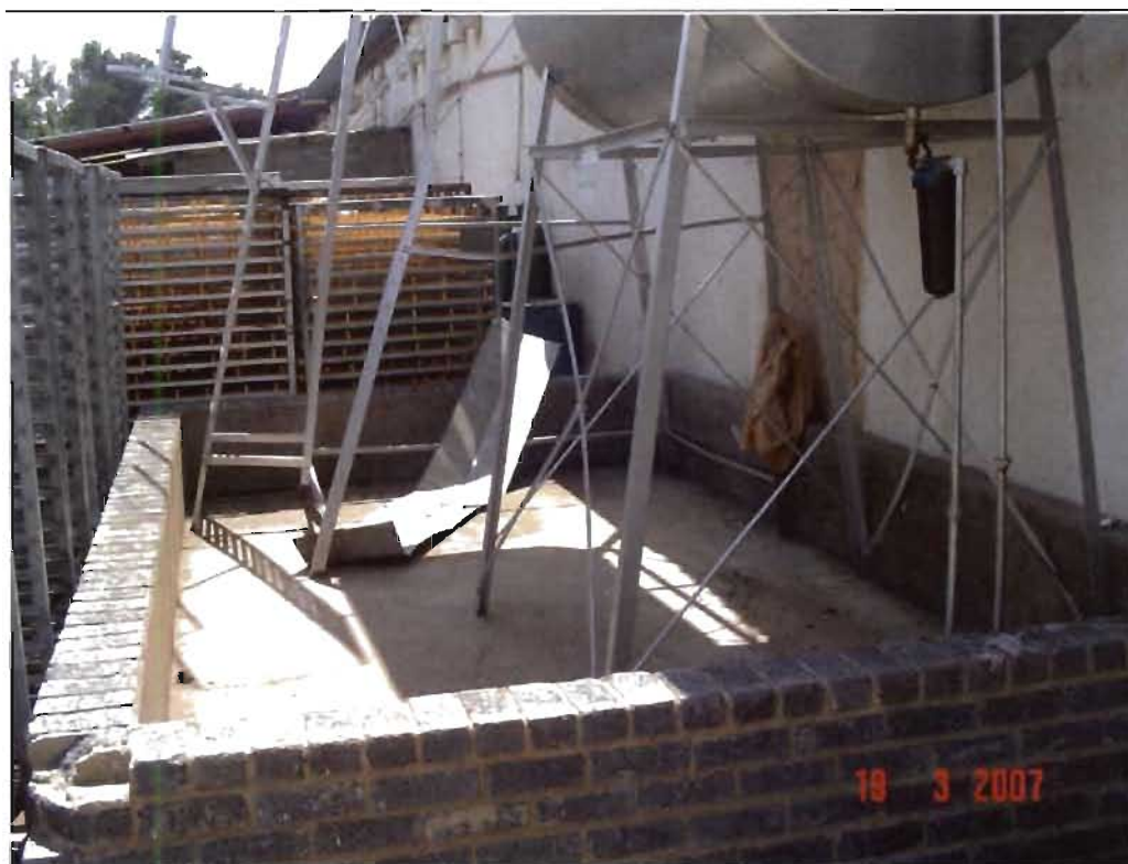
Photo 8.17 Site 3 – photo showing the condition of the tank bunding
