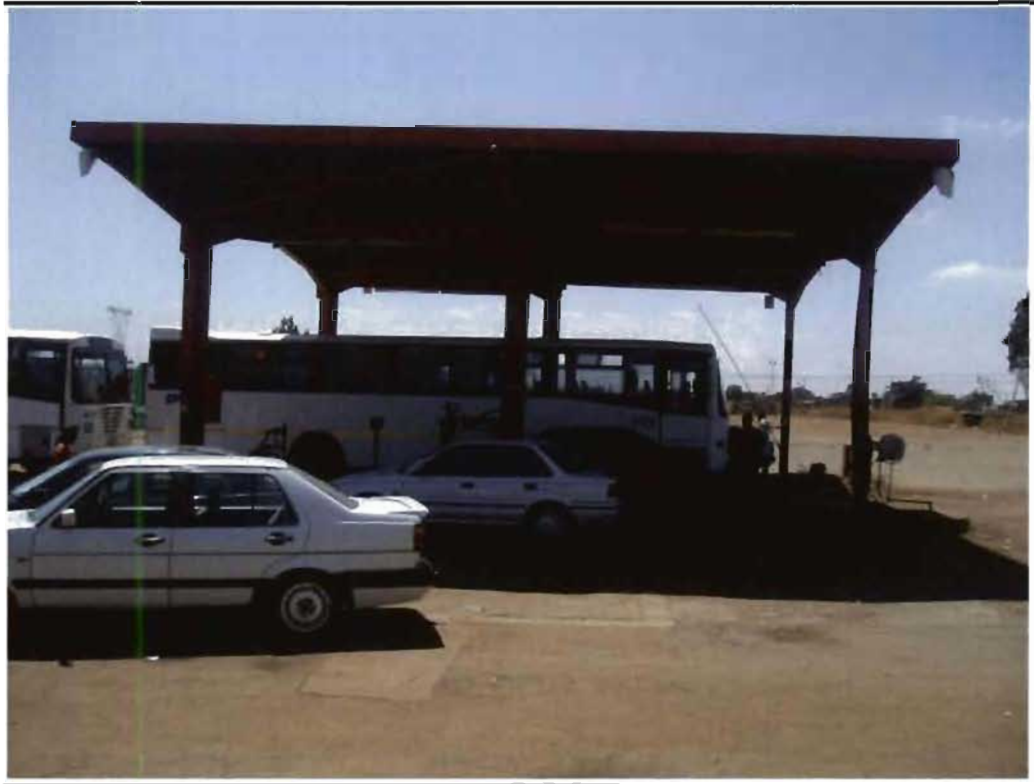
Photo 8.9 View of USTs from 10m looking north
