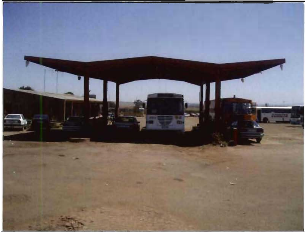
Photo 5.2.1 Location of the tank in relation to the bus servicing canopy looking north (S24/G/2/1023)
