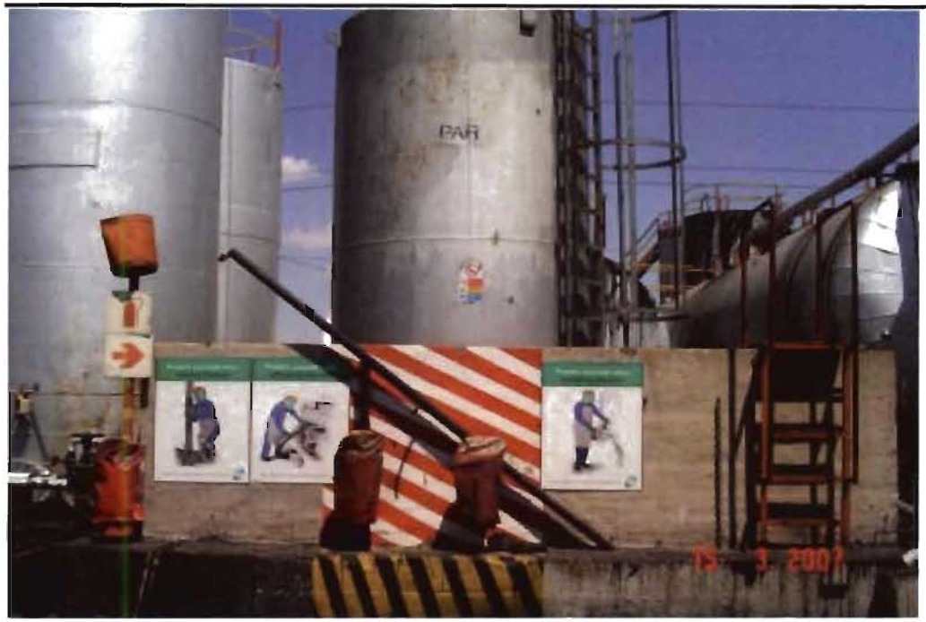
Photo 8.1 View of Shell-9,400 Litre AST, from 10m looking north
