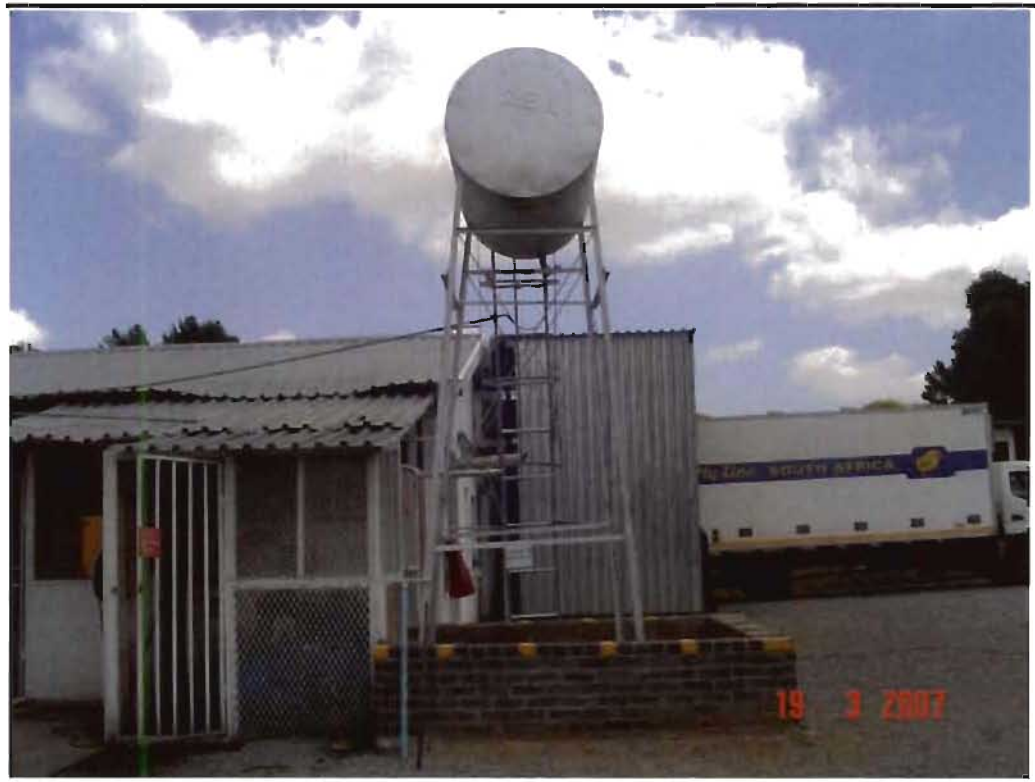
Photo 8.4 Site 1 - View of the tank from 10m looking east
