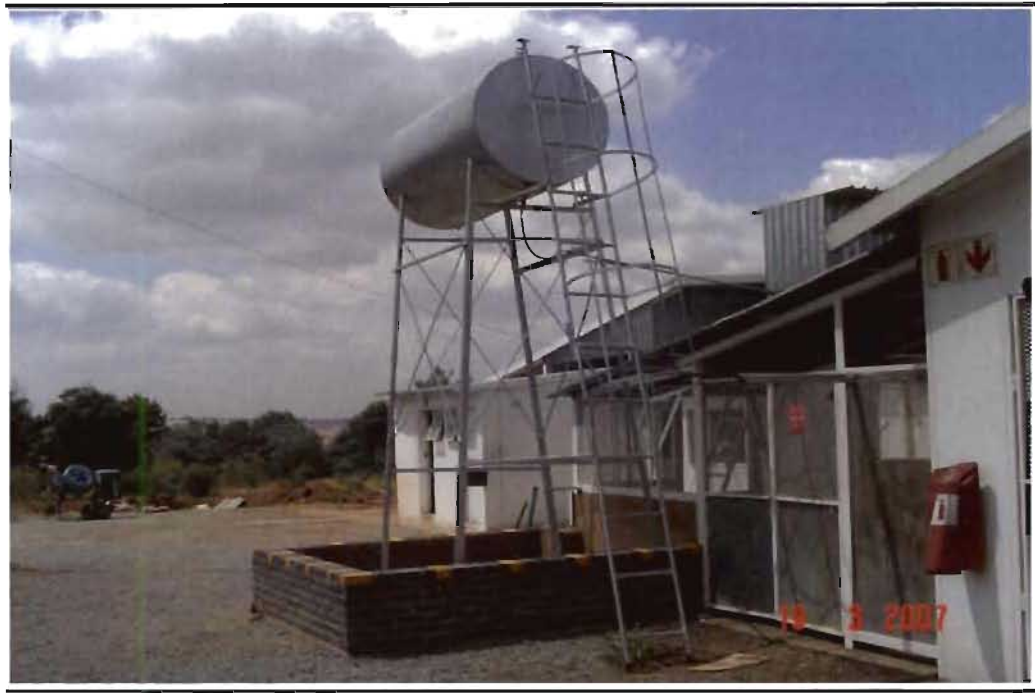
Photo 8.3 Site 1 - view of the tank from 10m looking west
