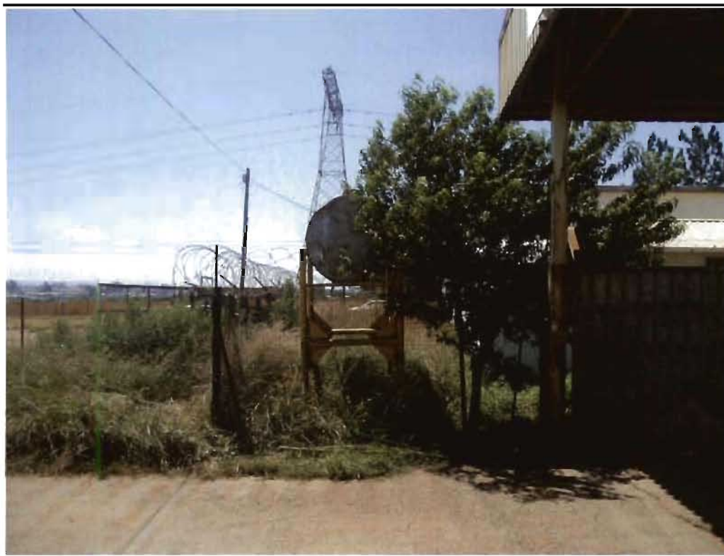
Photo 8.5 View of AST (tank 2) from 10m looking north
