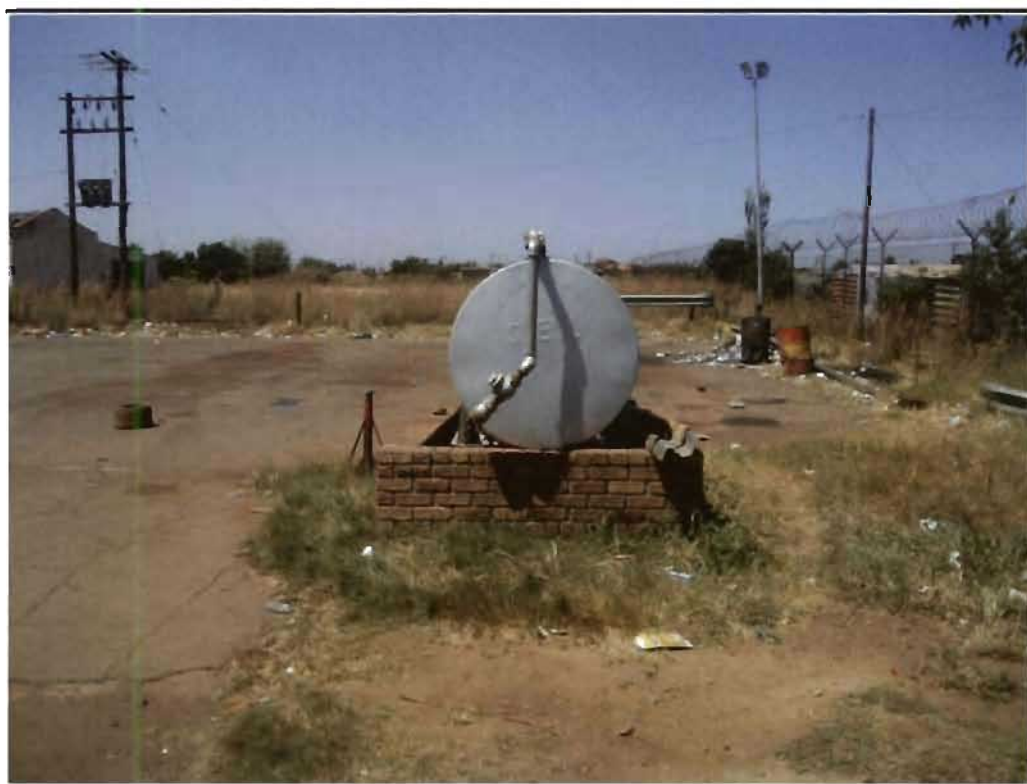
Photo 8.2 View AST (tank 1) from 10m looking east
