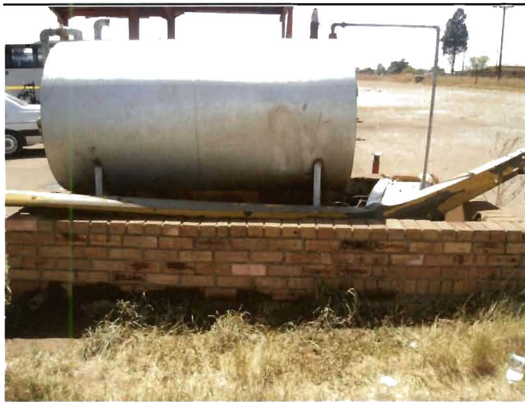
Photo 8.1. View of AST (tank 1) from 10m looking north
