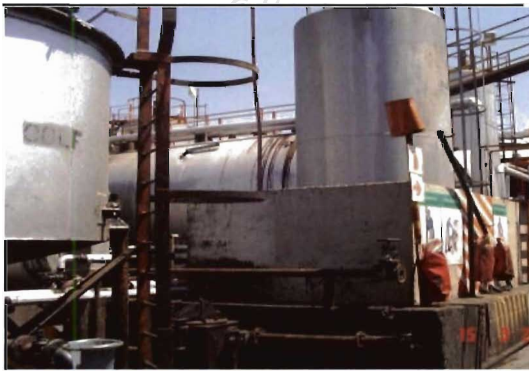
Photo 8.8 View of shell 9,400 litres AST, from 20m looking west
