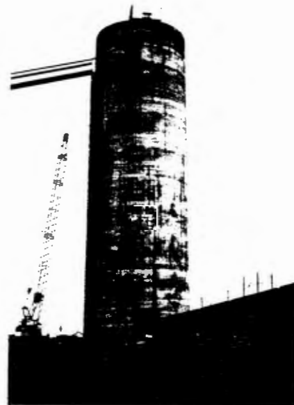
Figure 1: The Optimum Colliery load-out silos.
