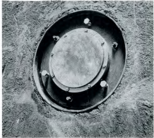
Figure 5b. Gauge installed in wall prior to grouting and smoothing off.
