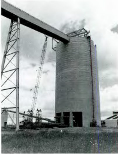
Fig. 4a: General appearance of 15,000 t run of mine coal bin
