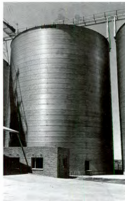
Fig. 9: 18.2 m diameter by 24 m high maize storage bin undamaged after eccentric emptying through opening at base (visible to right of photograph)
