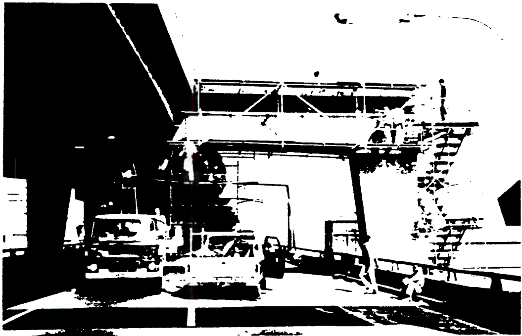
Figure 7: View of portal frame being prepared for full-scale load test
