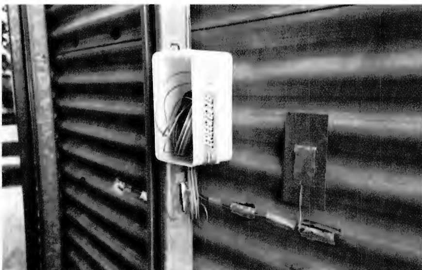
Fig. 3: Close-up of instrumentation on wall and stiffener of 12.5 m diameter silo
