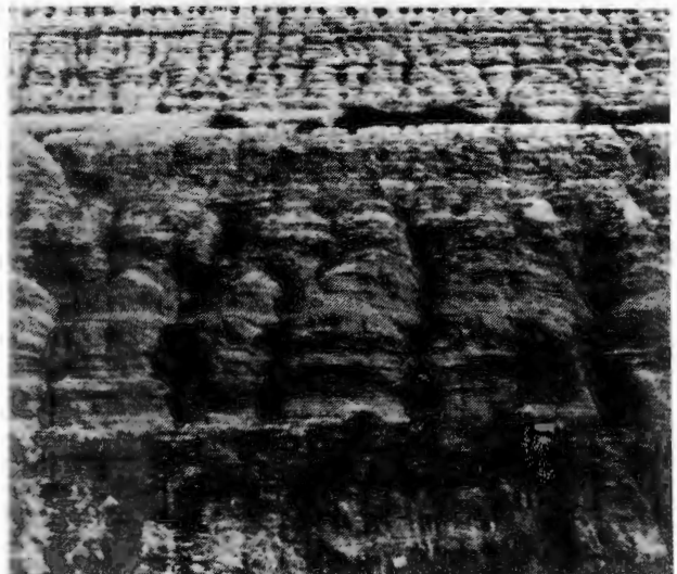
Figure 10 : Eroded surface of a gold tailings dam.
