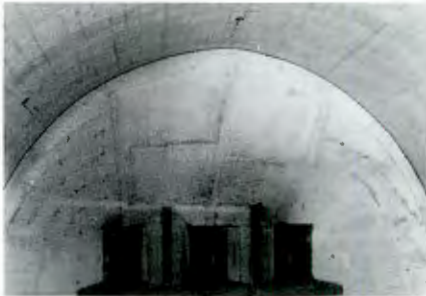
Fig. 4b: View into 15,000 t bin showing 3 of 6 outlets. Pressure cells are visible at 12 o'clock and 1h30 in photograph, on bin wall
