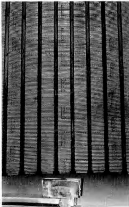
Fig. 1b: View of inside of silo showing stiffeners
