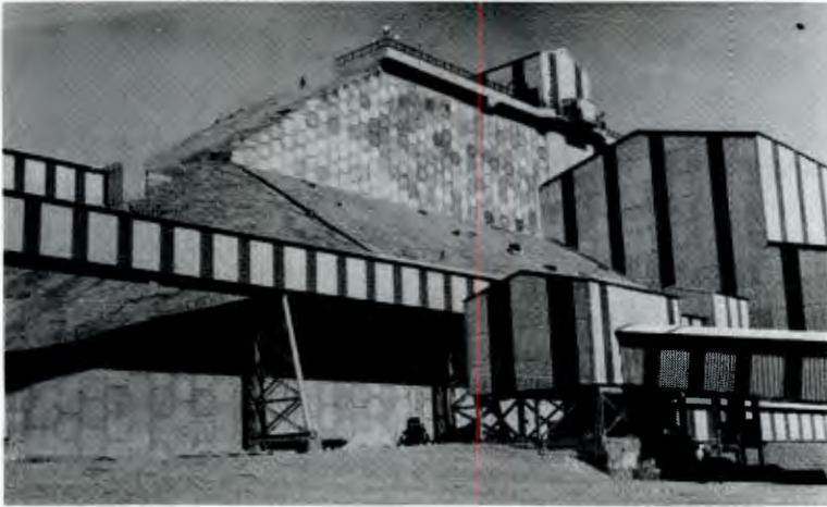
Fig. 2. View of reinforced earth walls H (above) and G (below)
