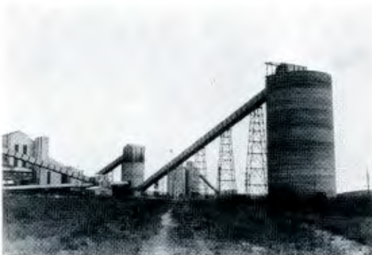
Figure 1(a). The coal load-out bin and associated plant
