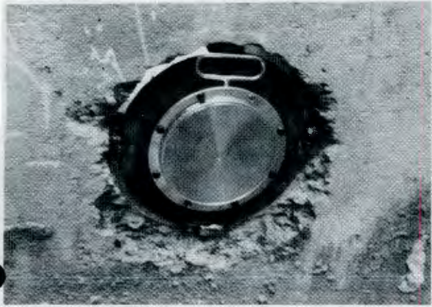
Figure 3(b). Typical pressure cell during installation.
