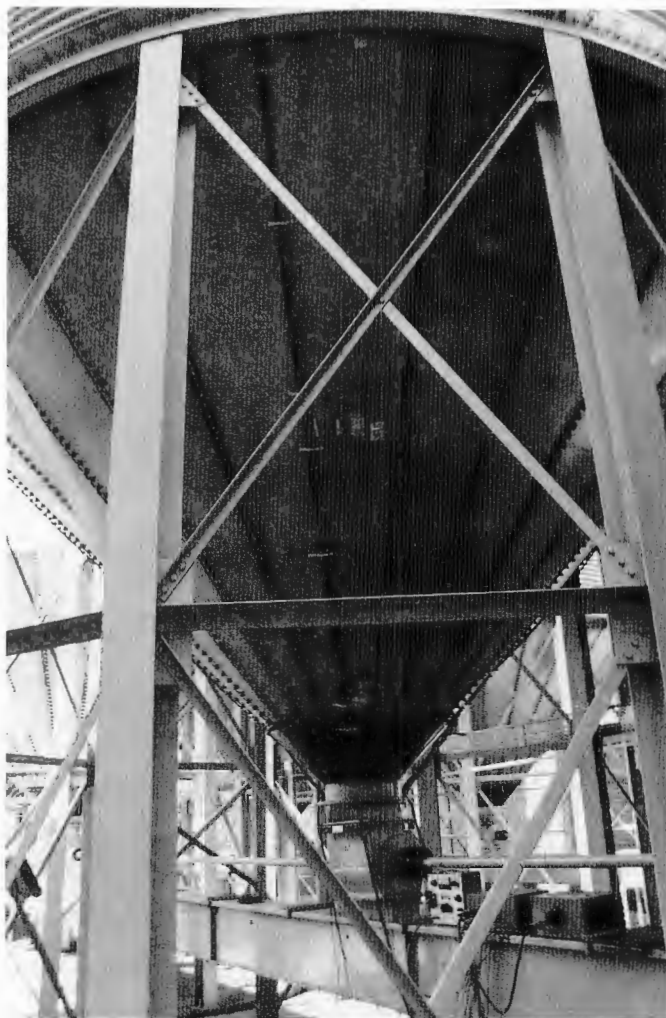
Fig. 3: View of conical hopper at base of test silo
