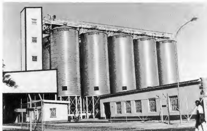
Fig. 2: View of silo complex at Bethlehem, South Africa
