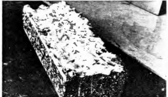
Fig 4: Thin layer of concrete adhering to underside of epoxy mortar nosing after disbonding failure
