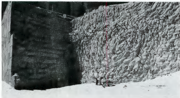
Fig. 13. Excavation on wall A—15 m high
