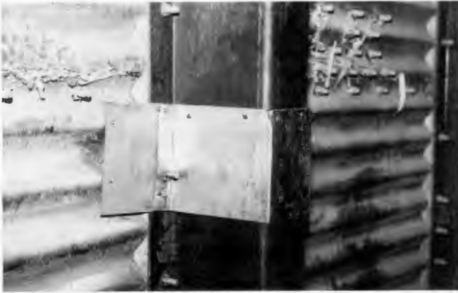
Fig. 3a: Steel sheet protecting strain gauges on internal stiffener
