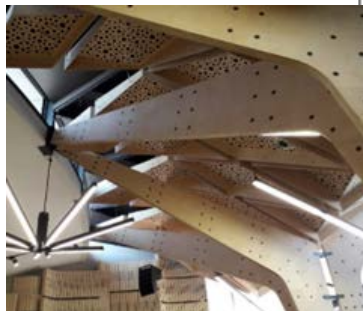
Figure 45: Plywood portal frames in the conference centre.
