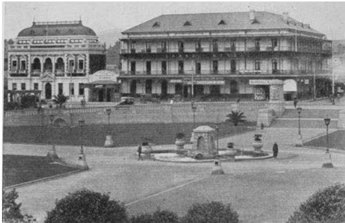
Figure 77: The second fountain in the centre of Church Square around 1929, with the southern entrance to the right in the background. From Van der Vyver EY.
