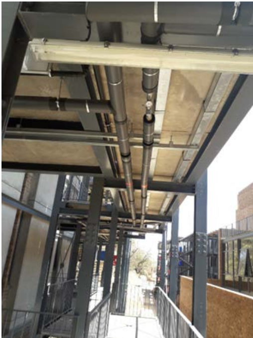
Figure 32: Housing units passage. Image by Author.
