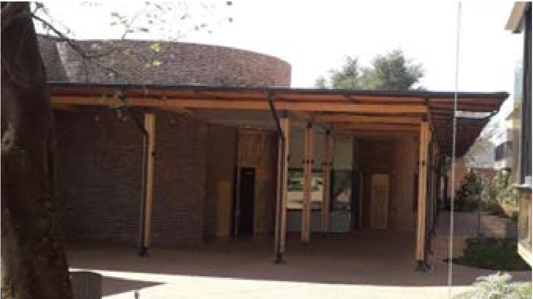
Figure 30: Future Africa Campus Conference Facility. Image by Author
