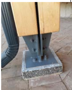
Figure 44: Timber column footing.
