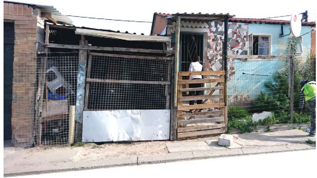
Figure 51: The use timber as structure and support and cladding in Delft
