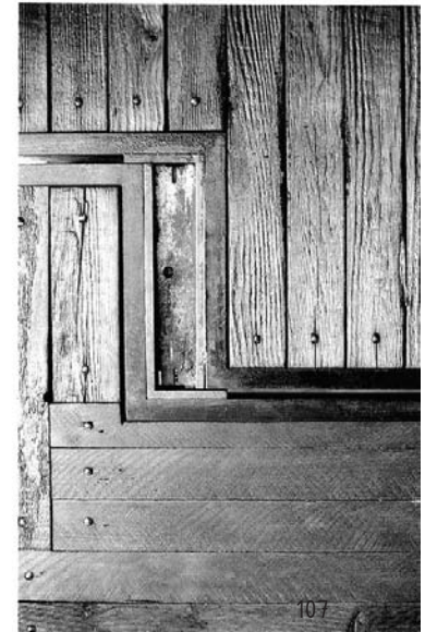
Figure 50: New technologies and techniques suggested, a combination between steel and timber. Carlo Scarpa 'Joint'
