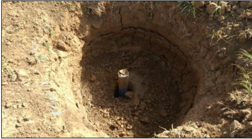
Figure 2-1: Temporary borehole used for irrigation using the pumping machine at Shinaka Fadama site.
