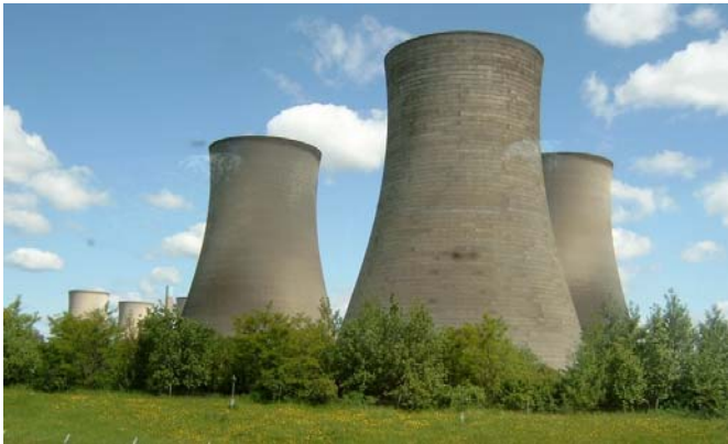
Figure 1: Picture of hyperbolic cooling towers adopted from ( http://en.wikipedia.org/wiki/Ferrybridge-power_stations , n.d.)
