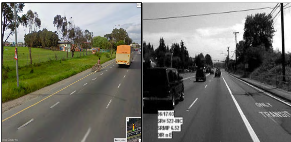
Figure 3-31 Lansdowne Road Shoulder near Jan Smuts Road, Cape Town intersection (courtesy of Google Maps) and a BBS in Washington State, USA (Lee et al., 2006).
