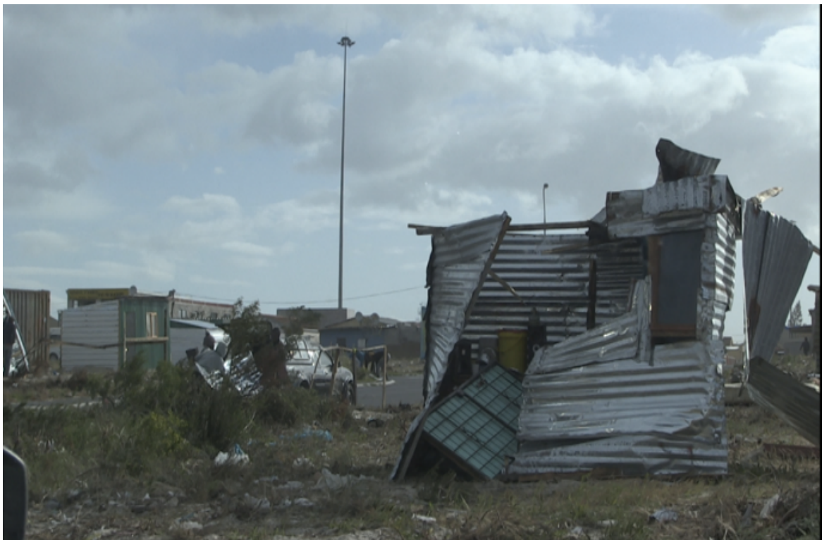
Figure 27: Shacks being demolished by strong wind (Photo by Minga, 3 December 2020).
