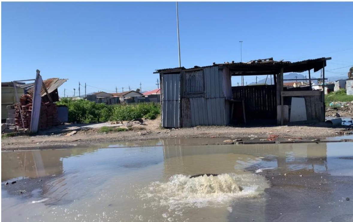
Figure 17: Evidence of overflowing drains on the street (Photo by Minga, 19 September 2020).
