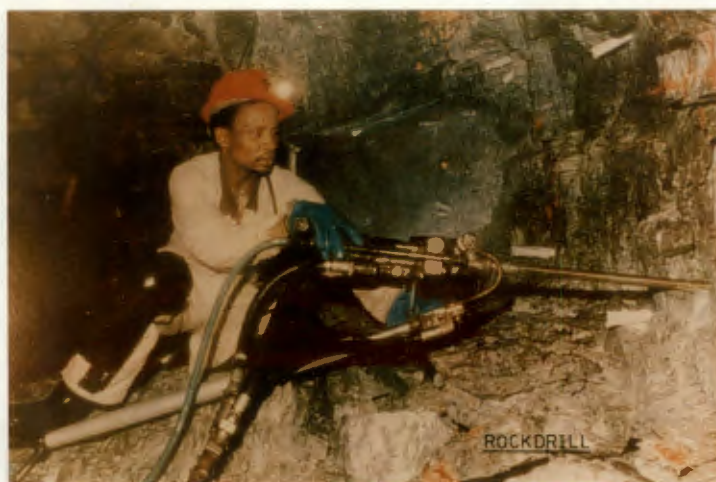
Fig. 1.4 ROCKDRILL IN OPERATION UNDERGROUND
