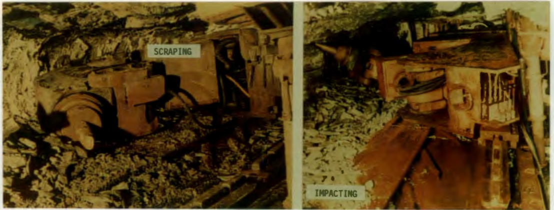
Fig. 1.2 IMPACT ROCK BREAKING MACHINE IN OPERATION UNDERGROUND
