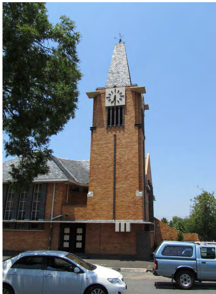
Figure 64 The former Johannesburg West NGK, a constant in the changing environment of Mayfair West.
