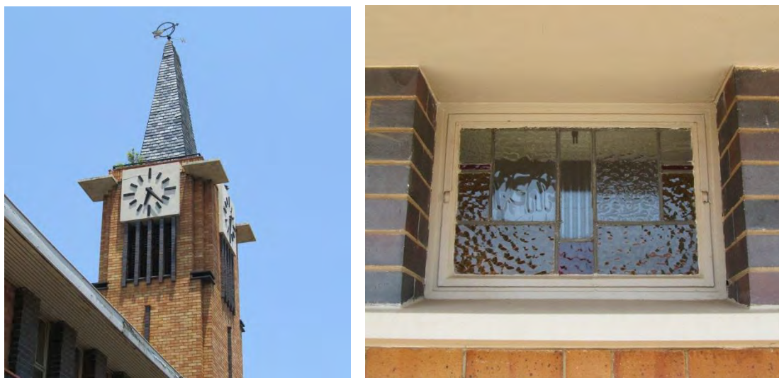
Figures 53-54 Details of the Steeple and stained glass windows
