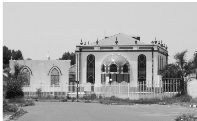
Figures 41-43 The Transvaal Mosque in Johannesburg Clockwise from left: the old Juma Masgied, 1918, now demolished (Le Roux 1994:20); The old Hamidia Mosque, Newtown, 1906, now substantially altered (Itzkin 2001:54); The 23 rd Street Mosque Pageview, the last remaining Transvaal style mosque in Johannesburg.
