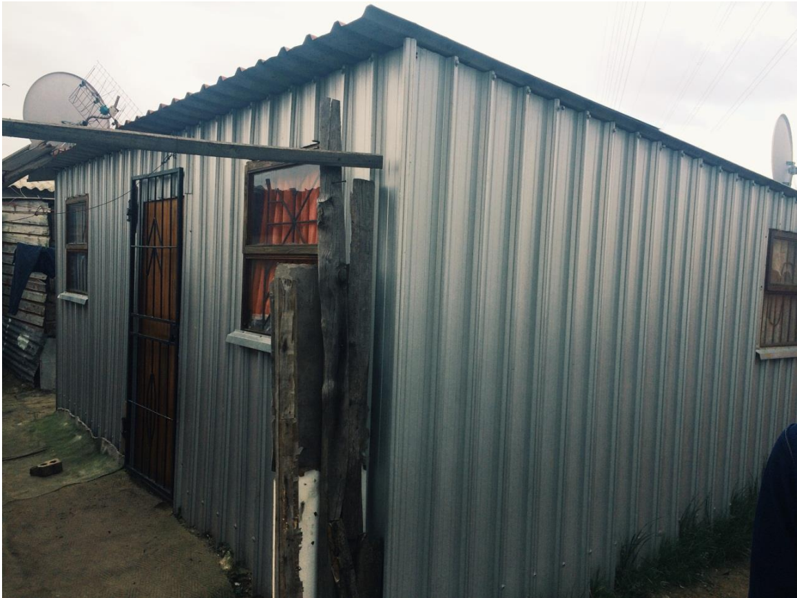
Figure 3 – Upgraded Ikhayalami shacks
