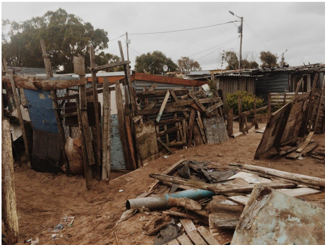
Figure 2 – Typical shack dwelling in Khayalitsha Township
