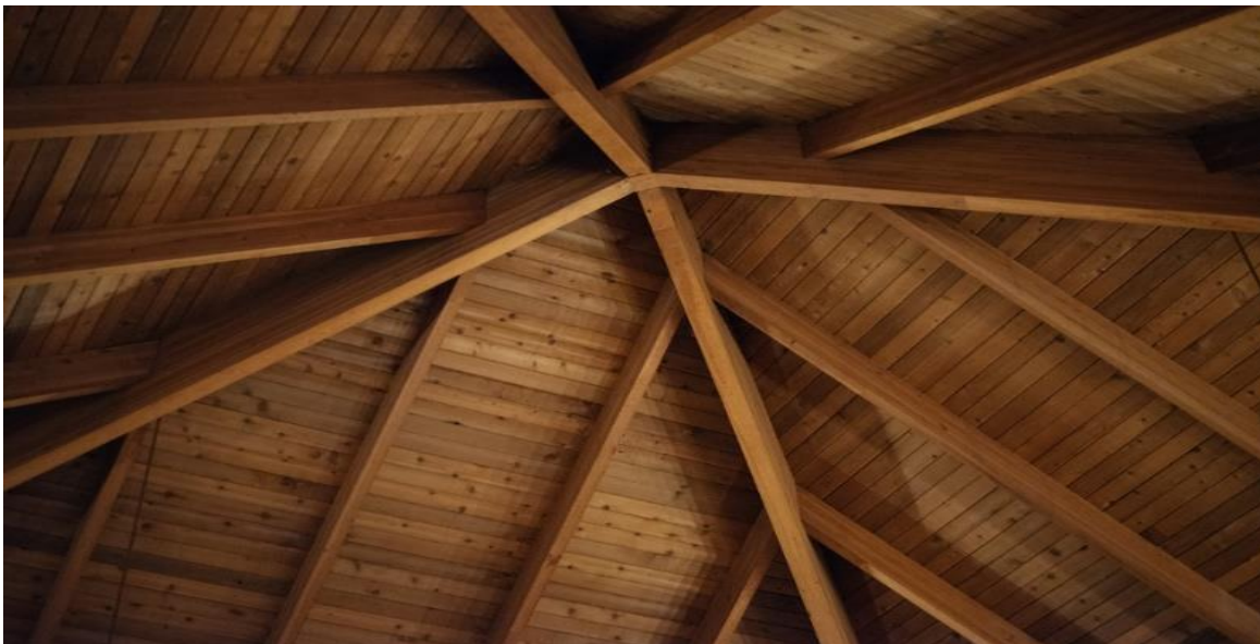
Figure 22. Douglas fir arches supporting the studio ceiling. Source: Construction of Englewood Cliffs – RVG Legacy, n.d. Photo credit: Atane Ofiaja.
