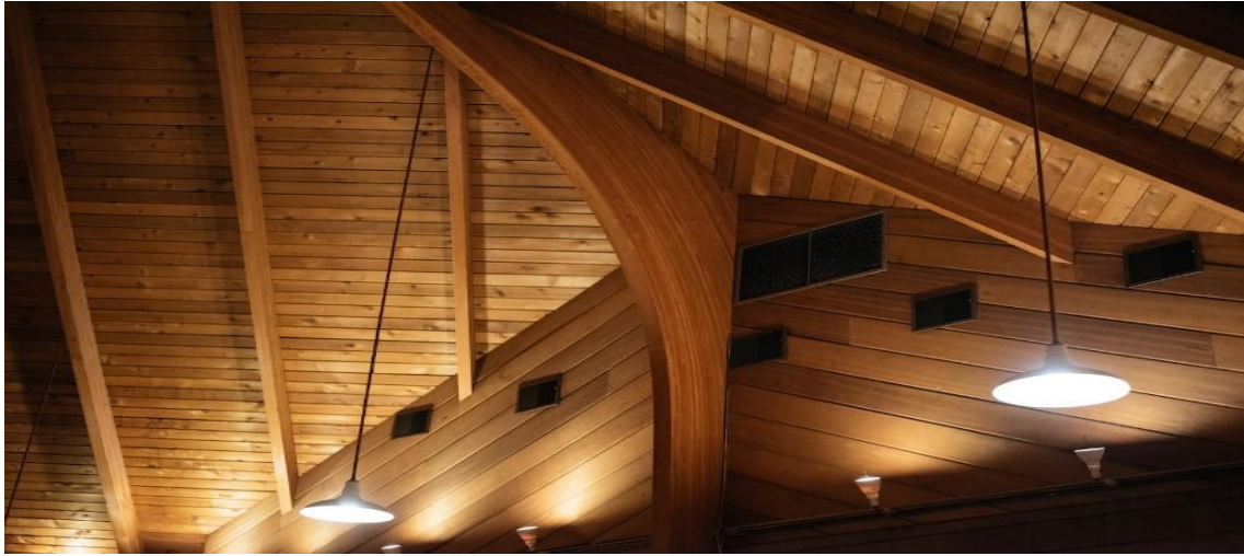
Figure 22. Douglas fir arches supporting the studio ceiling. Source: Construction of Englewood Cliffs – RVG Legacy, n.d. Photo credit: Atane Ofiaja.
