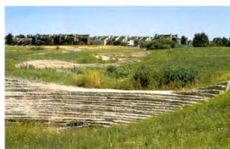
Figure 3.56 Drop structures in the wet season (source: Margolis, L. et al 2007)
