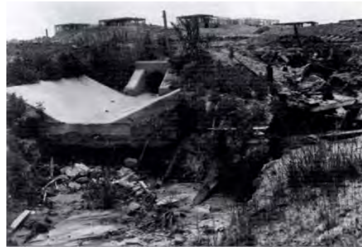
Figure 8.86 Slope erosion resulting from alteration of drainage, vegetation and soil associated with residential development. Bioengineering techniques are aimed at mitigating on such landscape destruction (source: Marsh, M.W., 1998)
