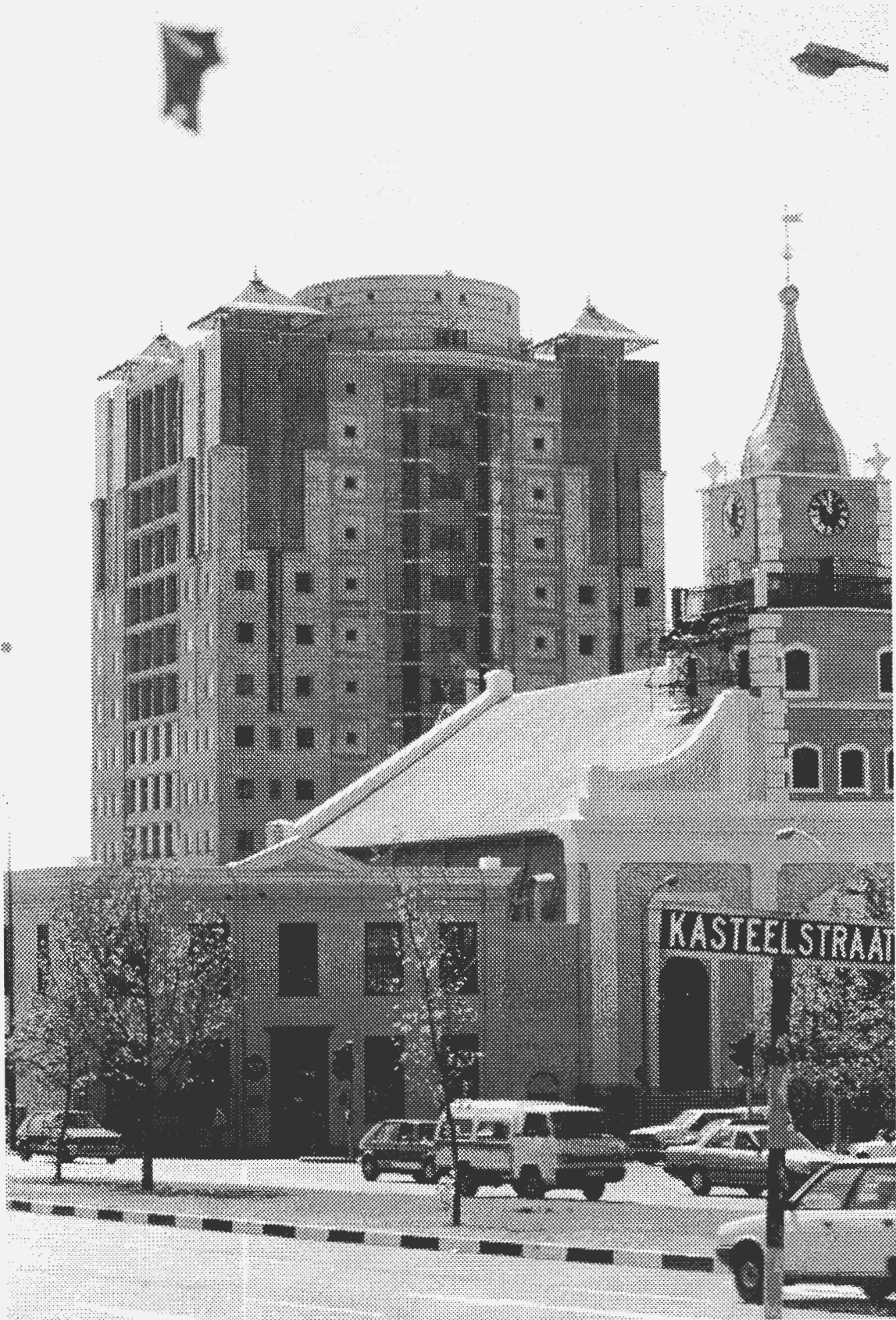
The Terraces: the Lutheran Church with the Terraces tower behind it (photograph 1994)
