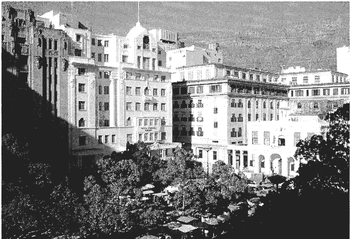
The Protea Building with its new extension overlooking Greenmarket Square (photographed in 1994)
