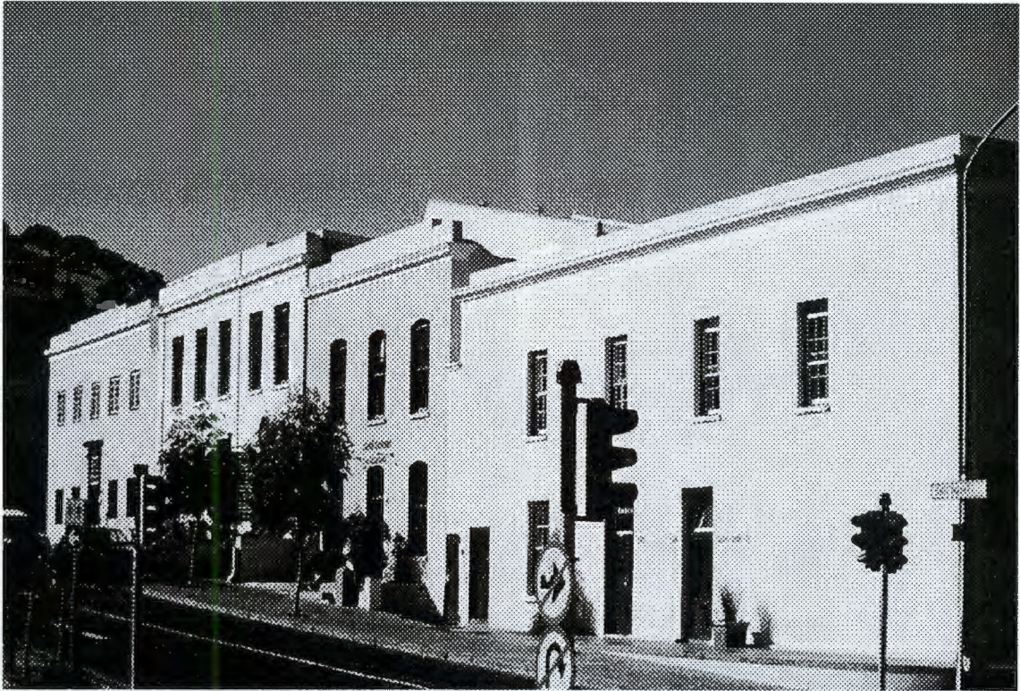
Heritage Square today: view up Shortmarket Street; the balcony has been removed and the Mourners' Chapel has been remodelled as a 19 th century residential building (photograph 2003)
