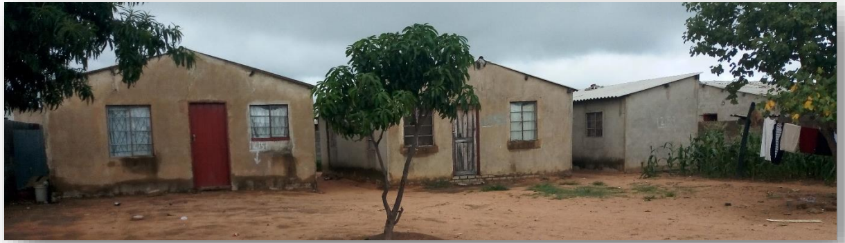
Figure 6-22: Typical housing in Housing Development 4
