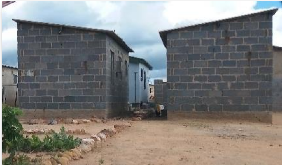
Figure 6-16: Typical housing in Housing Development 3
