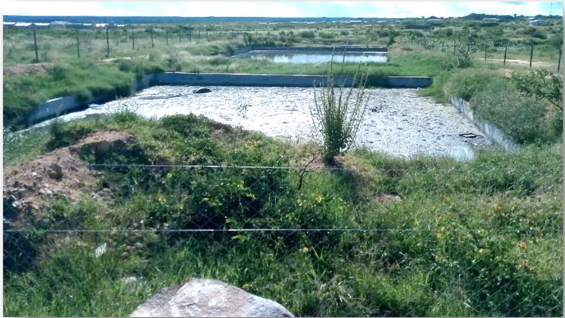
Figure 6-20: Sewer ponds in Housing Development 3
