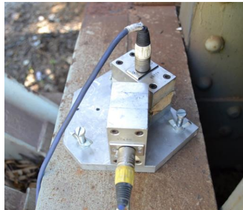
Figure 15: Image of accelerometer pair
