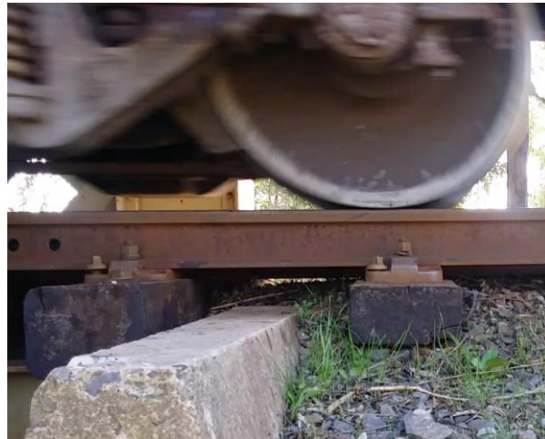
Figure 23: Image of rail line at the approach abutment
