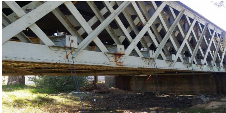
Figure 16: Image of actual positioning of accelerometers on site
