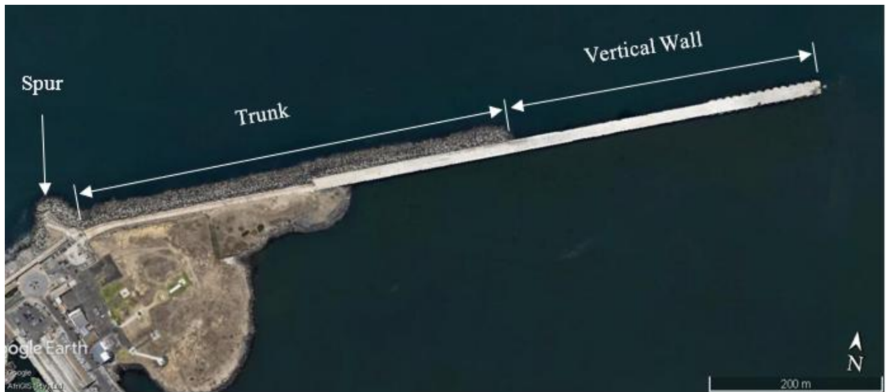
Figure 4.2: Port of Cape Town's Main Breakwater (Picture supplied by TNPA)
