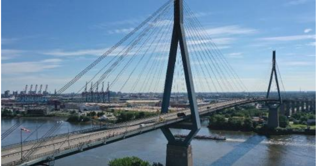
Figure 2.15: The Köhlbrand Bridge in Hamburg, Germany (Wenner, et al., 2021)
