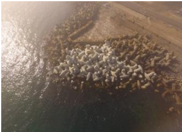
Figure 2.1: Table Bay breakwater at the Port of Cape Town (Picture supplied by TNPA)
