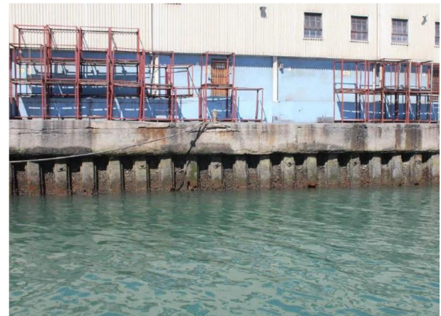
Figure 2.2: Sheet pile wall at the Port of Port Elizabeth (Picture supplied by TNPA)
