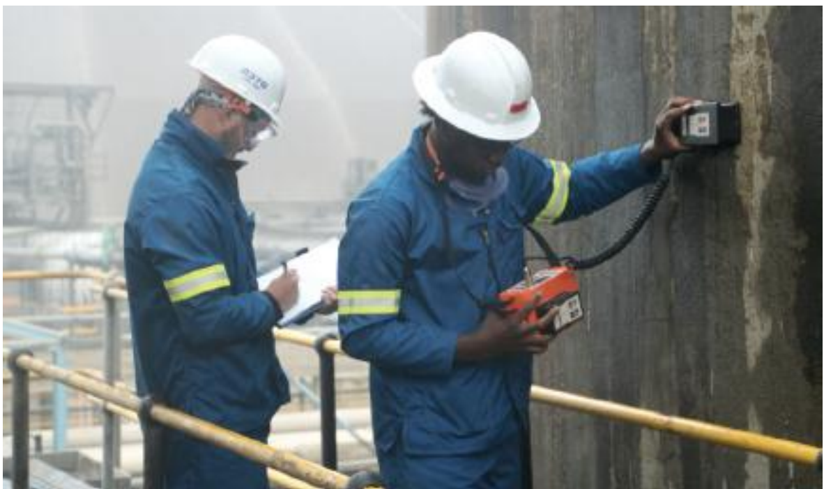
Figure 2.9: Cover depth assessment on site (Beushausen & Louw, 2021)
