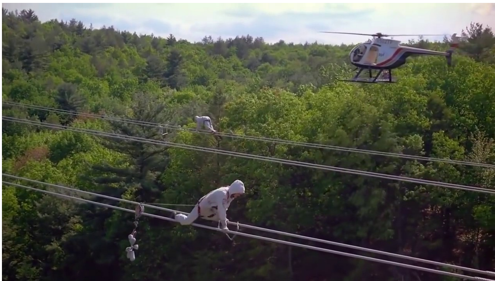
Figure 1.1: Image showing two men performing high-voltage live-wire inspection and maintenance at a high altitude [55]
