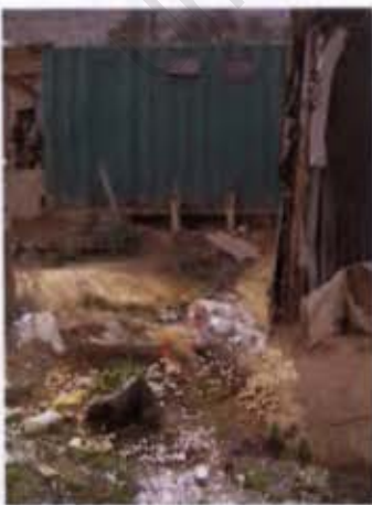
G: Langrug, leaking communal facilities
