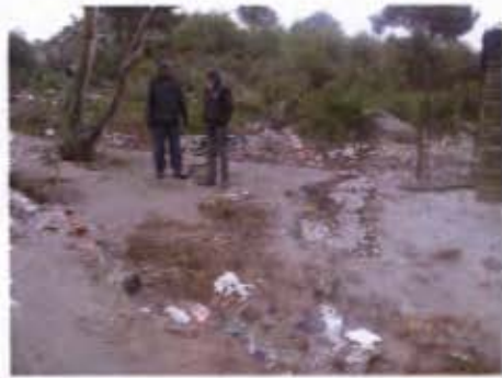
X: Waterworks, streams of waste water from sewerage line
