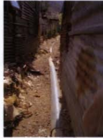
O: Langrug, residents waste water intervention
