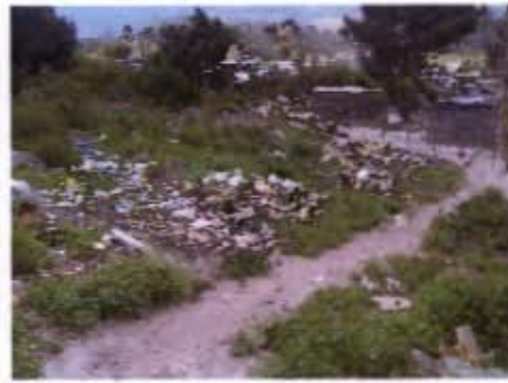
T: Waterworks, waste accumulation nearby leaking sewerage manhole
