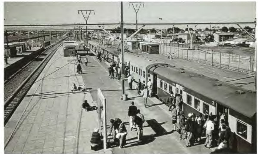
15. Metrorail Train Platform
