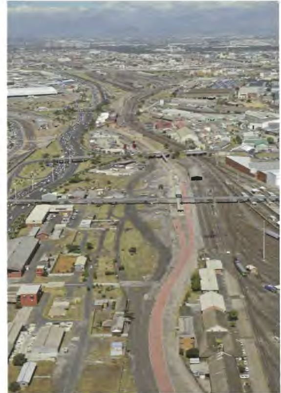
3. View looking to the north-east, including the site, rail lines, and N1 freeway.
