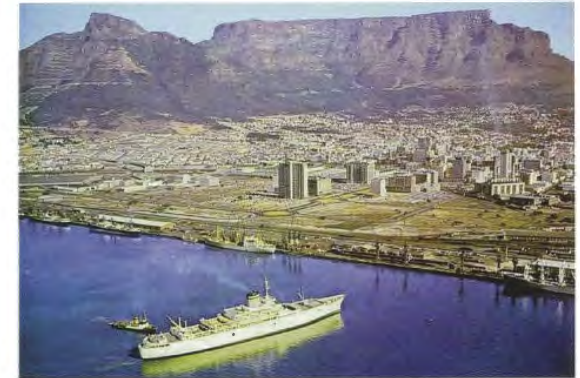
54. Construction of the Foreshore development begins on the reclaimed land.
