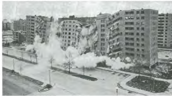
27. The demolition of Pruitt-Igoe in 1972
