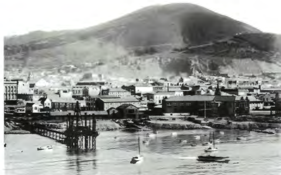
48. The working harbour before it was cordoned off from the city.
