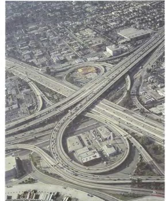
21 Infrastructure for the age of the automobile
