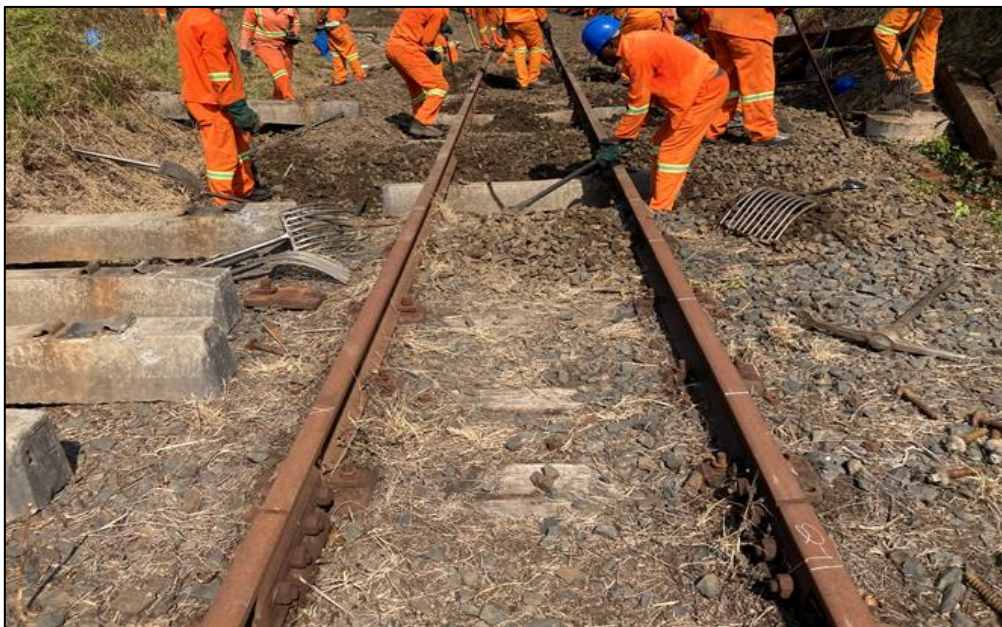
Figure 1.4: The replacement of deteriorated wooden sleepers with used concrete sleepers
