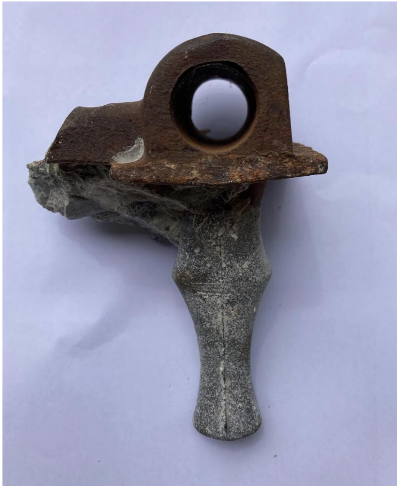
Figure 4.6: Condition of the cast iron immediately following extraction from concrete
