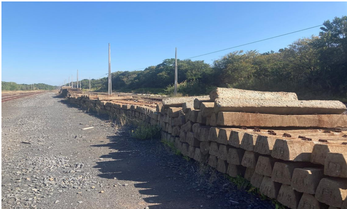
Figure 1.2: Stacked aged concrete sleepers removed from service; awaiting installation in the yard/station
