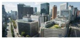
JR Osaka Station South Area An area blending global and local charms, with department stores, an underground shopping arcade, a hotel and more.
