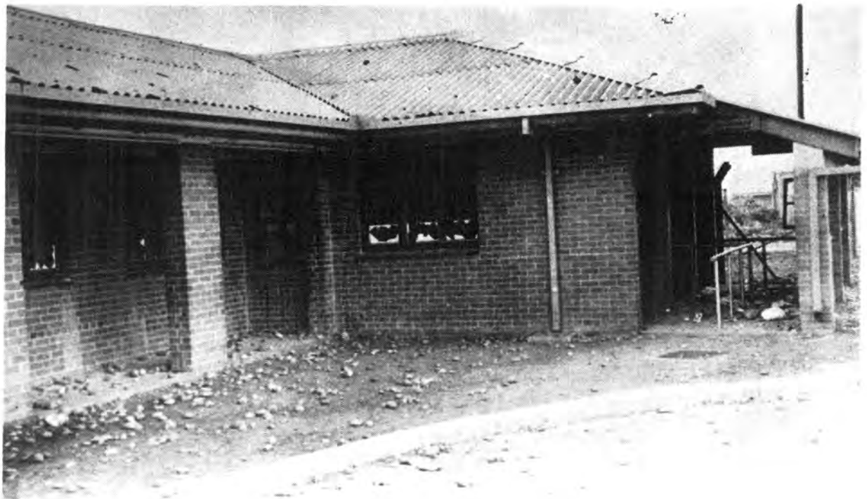
Illustration 9.1 New Brighton Railway Station Office after Stone Throwing, 18 Oct. 1952 (SAP Museum Archives, Pretoria).
