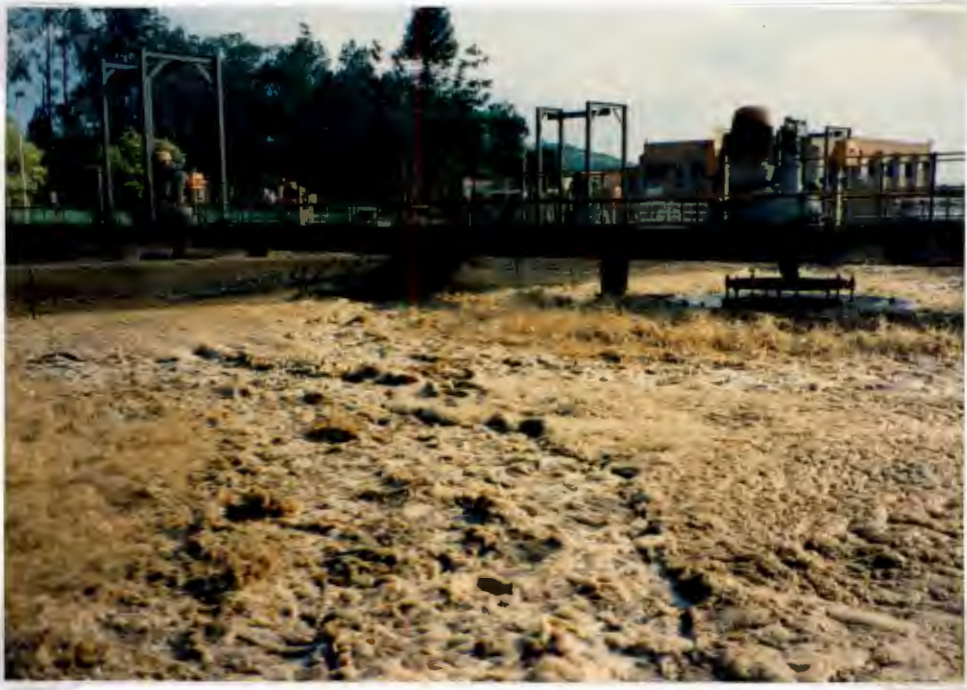
Photo 6.3: Nocardia -type foam forming in an aeration basin and accumulating between successive aerators.
