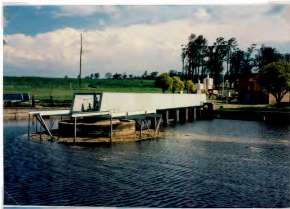
Photo 7.4: SST A showing scum trapped by the central skirt baffles and tending to carry-over into the effluent with the prevailing wind direction.
