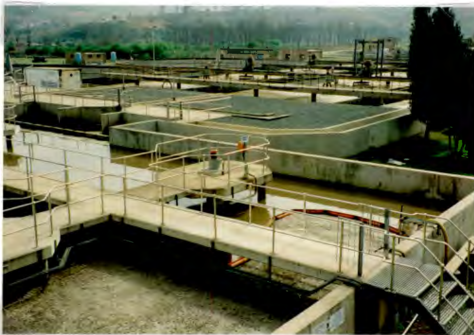
Photo 6.2: Anaerobic basin in foreground with Drizit ® floating boom in place during attempts to remove scum manually or using trash pumps.
