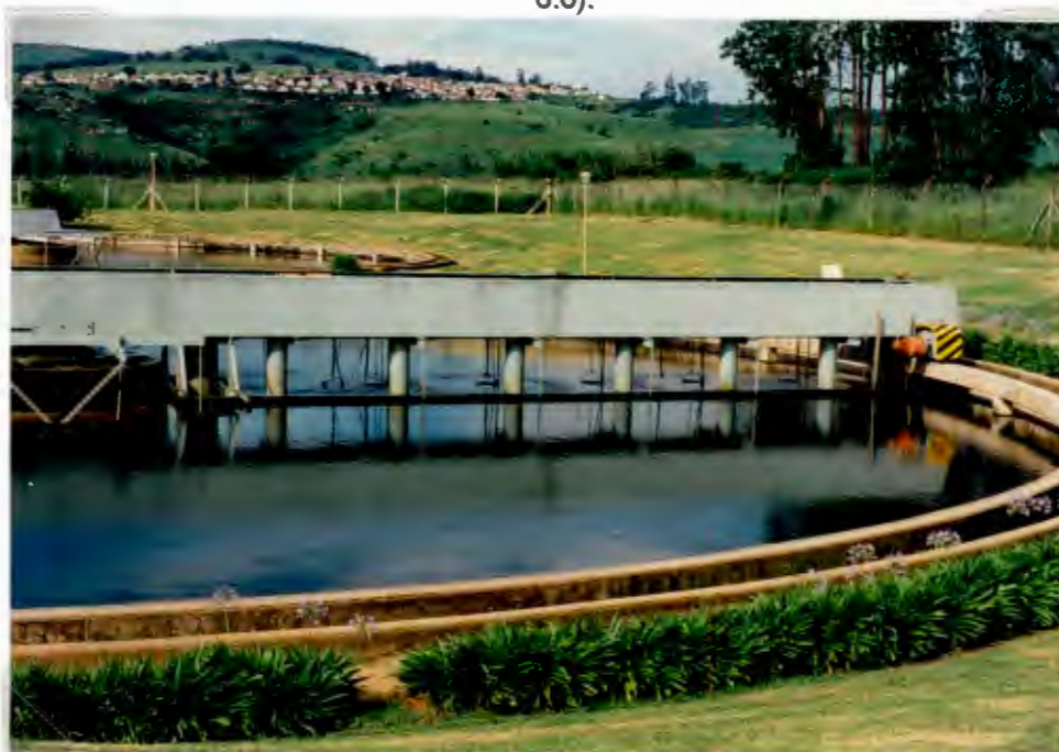
Photo 6.14: "Old" secondary clarifier (SST E) virtually free of scum on 14/1/97. Note: experimental water sprays were fitted as an experiment to this SST at the time of the Nocardia problem and may be seen here from the circular surface spray pattern on the far side of the clarifier bridge.
