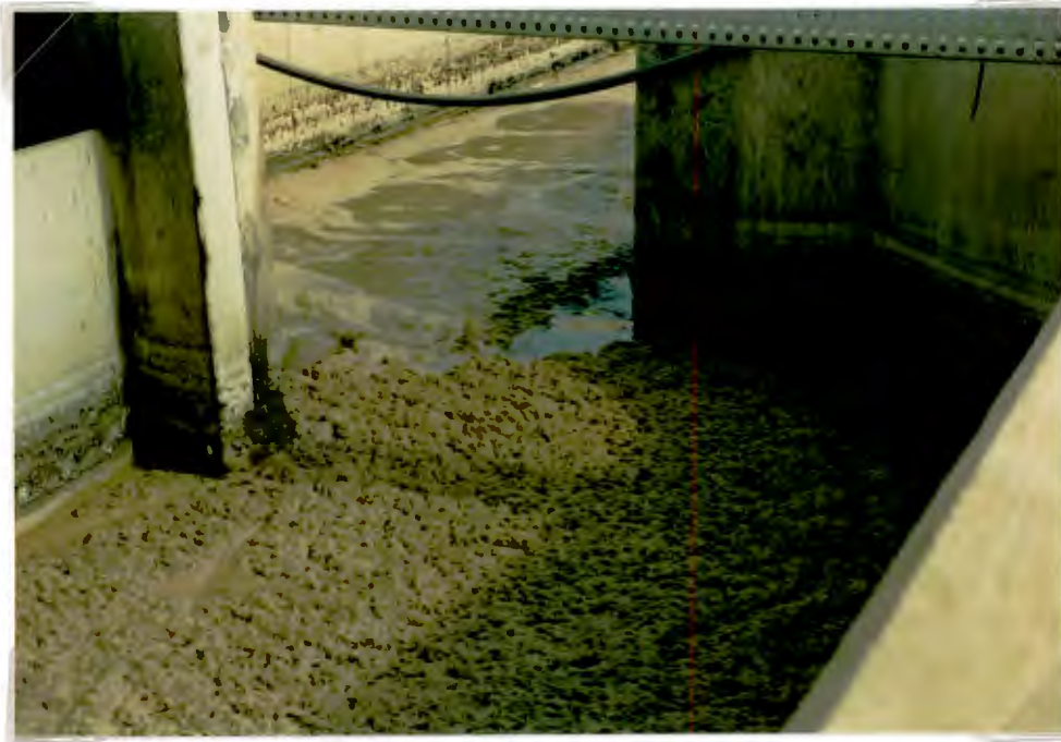
Photo 7.1: Nocardia foam/ scum travelling down channel from aeration basins to mixed liquor splitter box.
