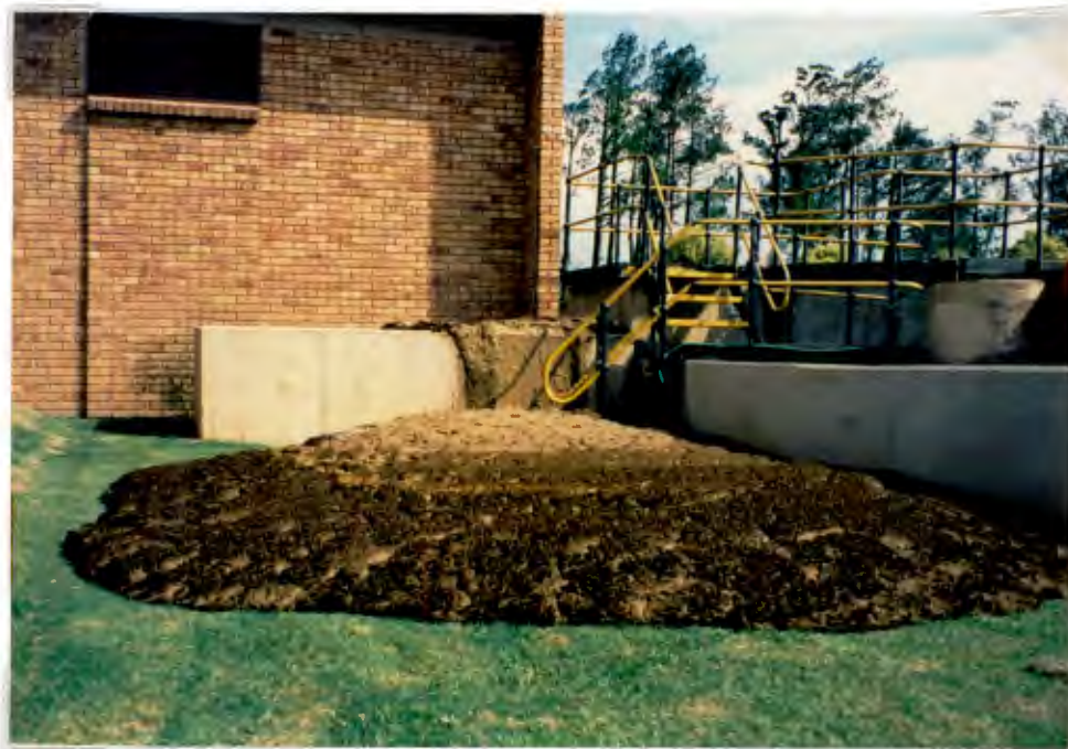
Photo 6.6: Foam emerging from junction box on mixed liquor pipeline to secondary settling tank. The foam created an eyesore and odour problem and had to be manually removed.
