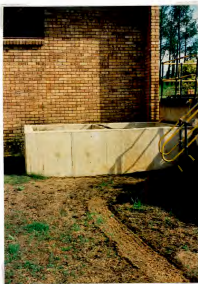
Photo 6.13: Junction box on mixed liquor pipeline to secondary clarifiers was completely free of foam on 14/1/97, six weeks after a resumption of alum dosing (compare with Photo 6.6).
