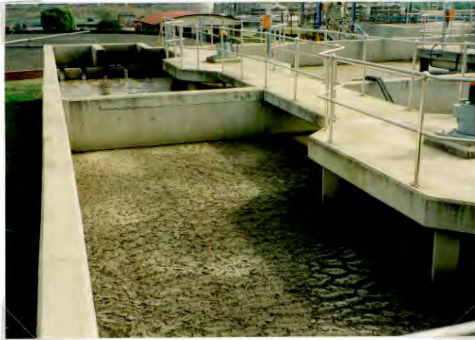
Photo 6.1: Anaerobic basin showing accumulation of scum. Whitish patches are granular HTH distributed on surface in an (unsuccessful) attempt to kill the Nocardia microorganisms.
