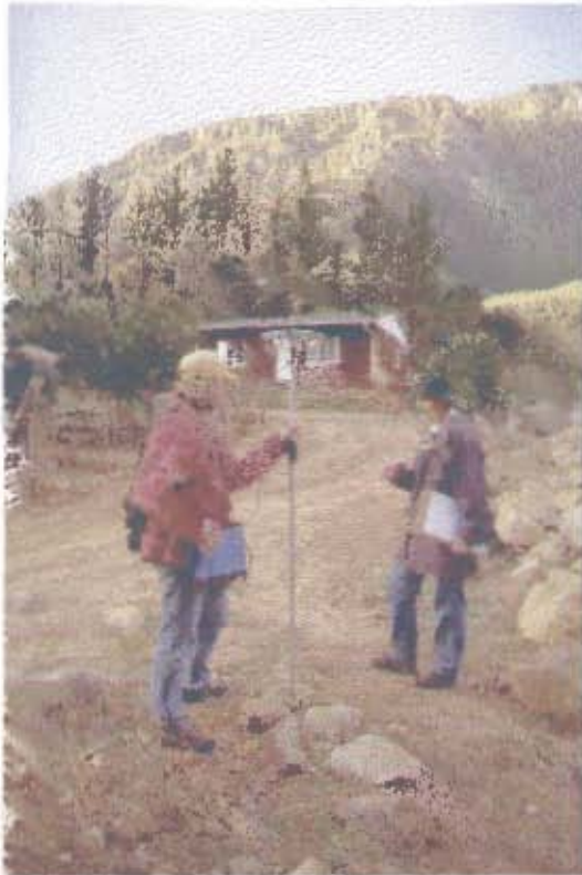
Figure 5.9: The GPS Survey in Bosdorp (Establishing a Base Station)
