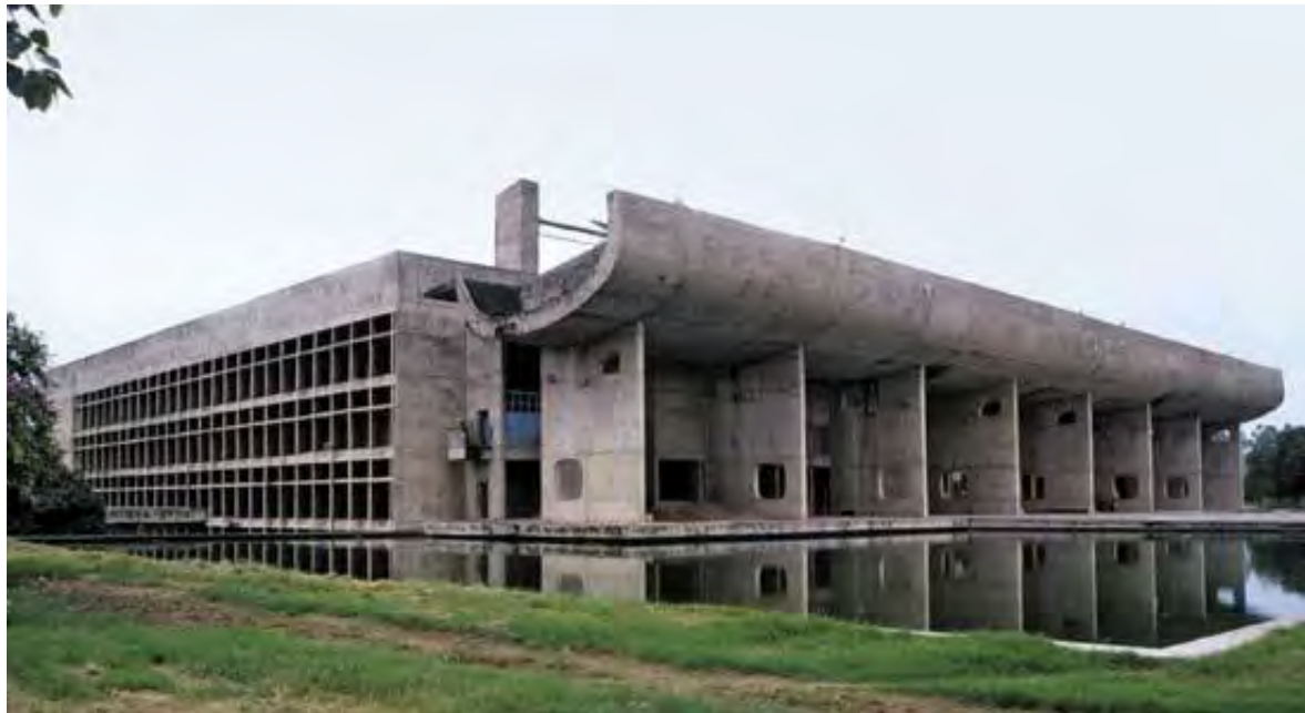
Fig. 13. Le Corbusier's Parliament building in Chandigarh, India. The form of the building celebrates the elastic qualities of reinforced concrete as most clearly indicated by the use of a massive, u-shape concrete roof that appears to be sailing over the entrance of the building. A clear expression of the building's massive structural elements on both facades gives it its monumental feel.
