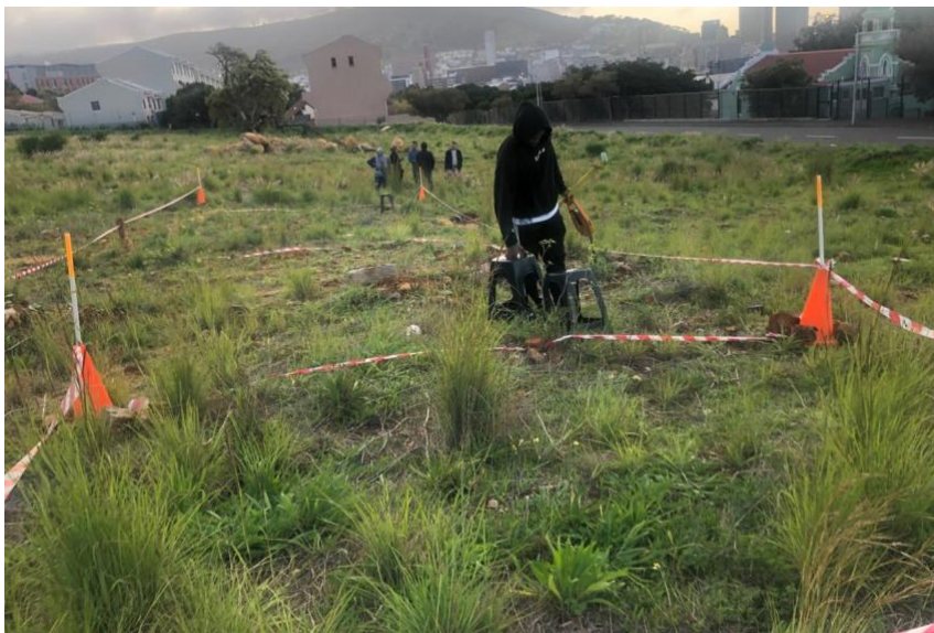
Figure 19: Site survey where the foundation of the house still exists
