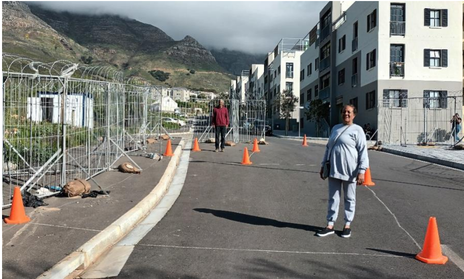
Figure 20: Site Survey where the foundation of the house has been removed
