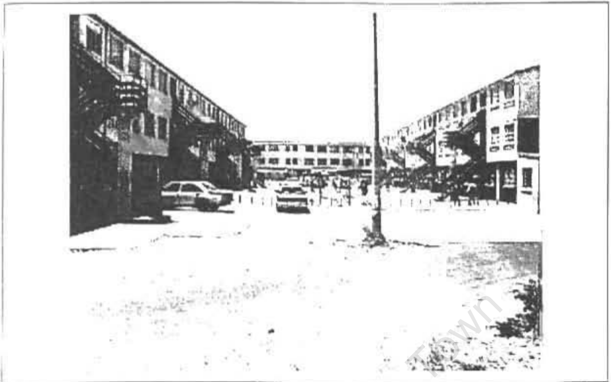
Plate 4.3 Invasion of privacy around staircases in Lavender Hill.
