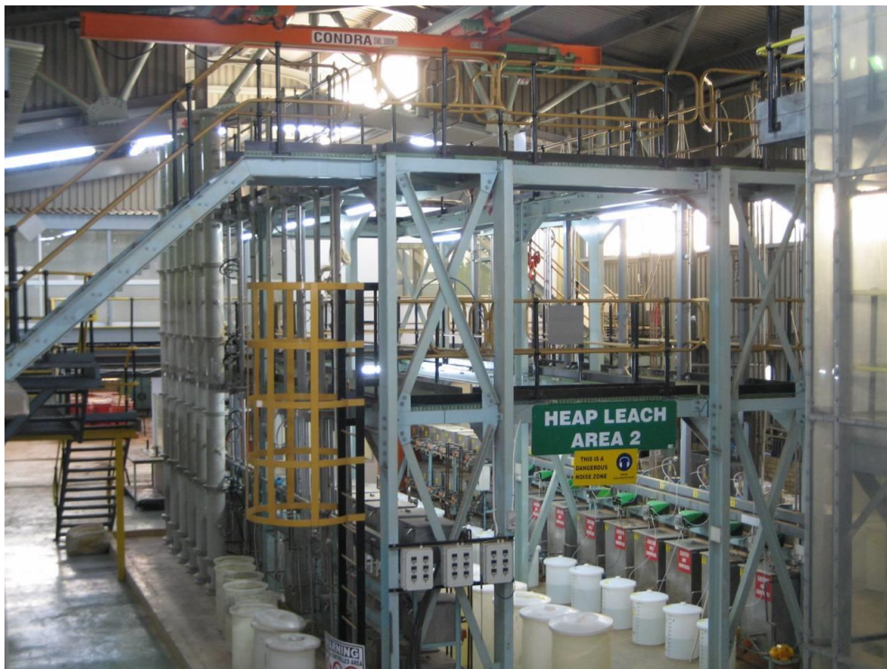
Figure 16. Tall column leach facility
