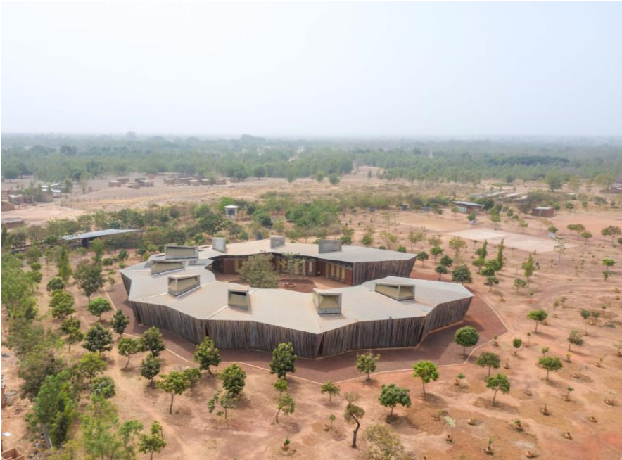
Fig 6.10: Roof tunnels The wind tunnels on the roof
