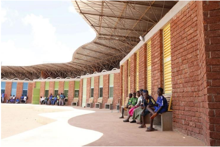
Fig 6.12: Gathering spaces Furniture is integrated into the walls of the buildings, creating comfortable places to sit shaded from the sun.
