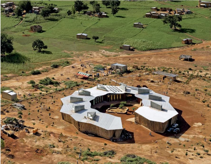
Fig 6.6: School aerial Aerial view of Lycee Schorge Secondary School.
