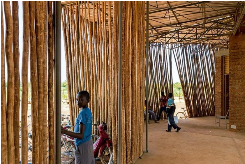
Fig 6.8: Timber screens The timber screen protect the passage from the natural elements.
