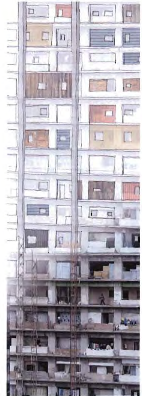
Right: Illustration imagining an architect's intervention in the Torre David skyscraper. The illustration shows a gradation for the skyscraper as it is today, into an imagined condition whereby an architect has established the fixes.
