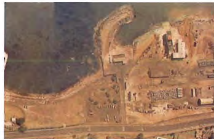
Figure 18 Aerial Photo showing rock base under reclaimed land at Granger Bay before Marina was built. Photo from PRDW engineers
