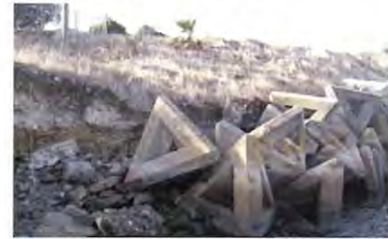
On site layers of rubble mound breakwater.
