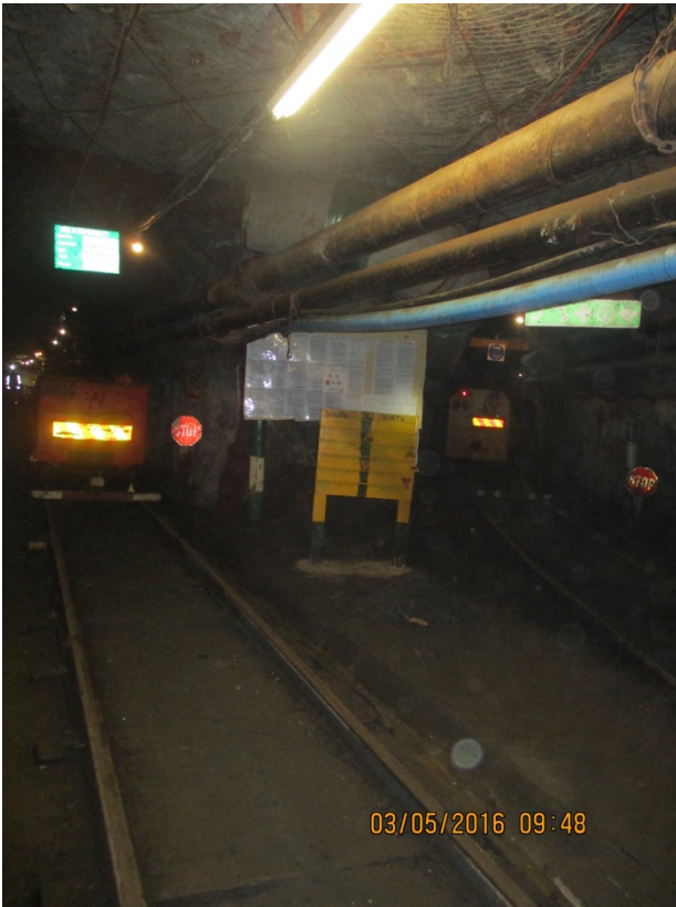
Photo 11: A typical tunnel underground
