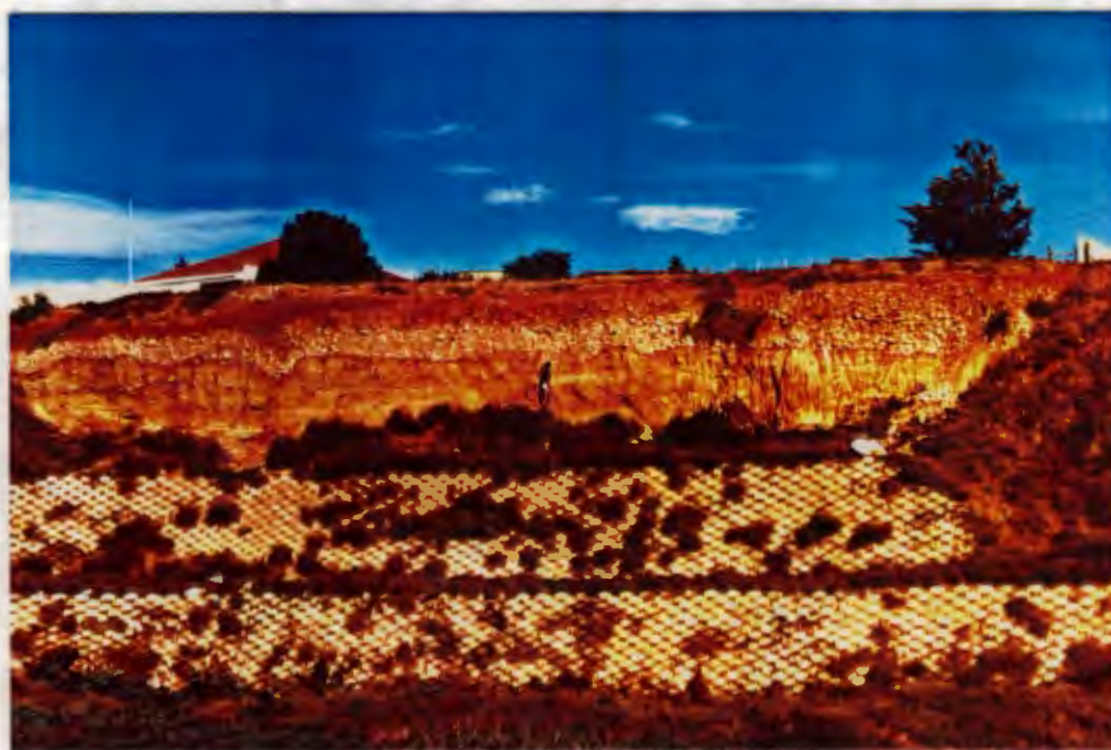
Plate 4: Fluvial terrace gravel deposit. View south from railway towards Genot Str. - Despatch. Note gravel filled palaeo-channels incised into semi-consolidated sandstone of the Sundays River Formation to far left and immediate right of figure.
