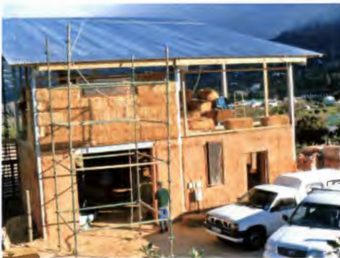
Structure built out of straw bales. (Green Building Elements, Images)
