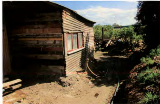
A drainage channel that guides water run-off from the highway away from this home.
