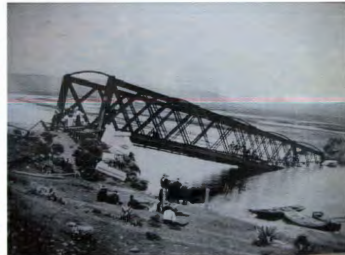
The railway bridge, crossing the Little Brak River, collapsed in 1905 because of floods. This serves as an example of how man-made structures fail if it is not designed with a good understanding of the landscape. (River Health Programme. State of River Report . p26.)
