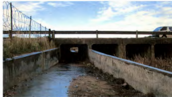
The existing, crawl-height, pedestrian subway
