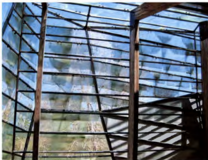
View of earth walls and roof structure. (www.cadc.auburn.edu. 2009)
