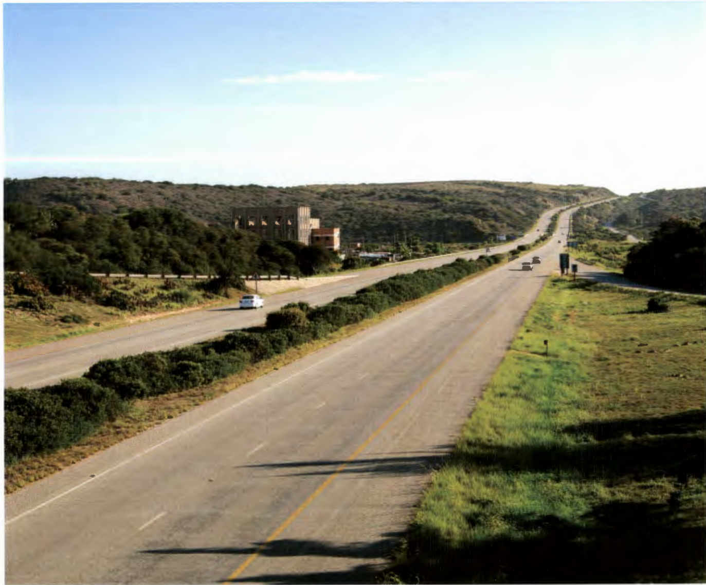
view of power town from the national highway
