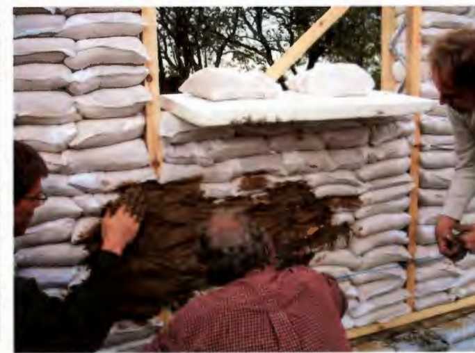
Sand bag house being constructed (Design Indaba, Images)
