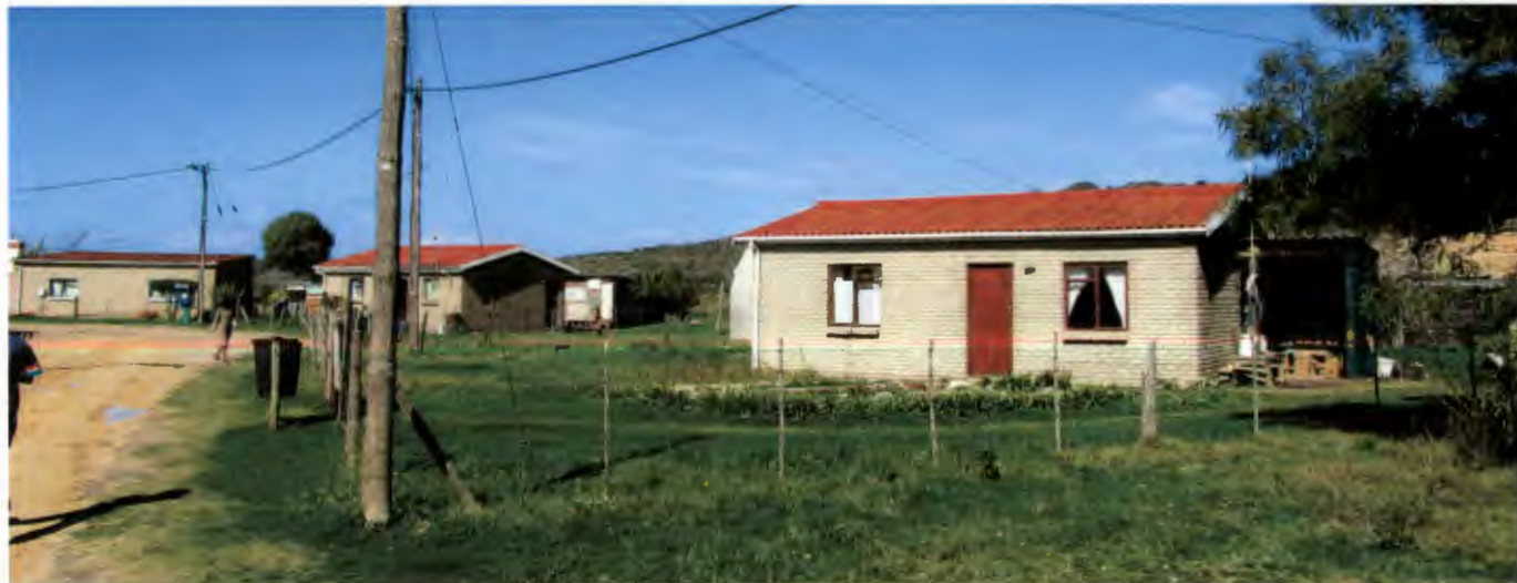
brick houses built by government for accommodation for water works employees
