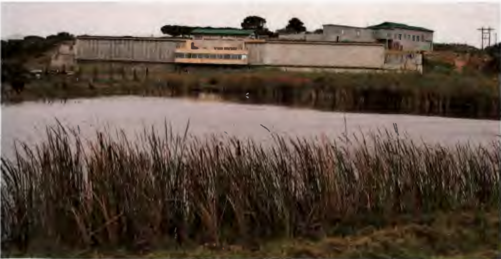
The water purification plant next to the town indicates the beginnings of a possible productive landscape
