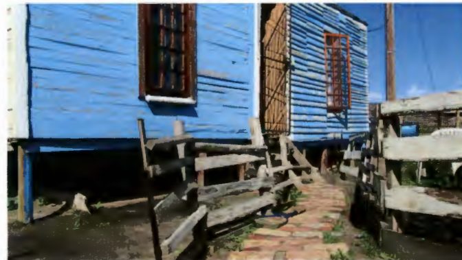
house built on stilts as an attempt to live above the flood line
