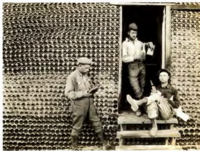
Discarded glass bottles used as building material. (Green Building Elements, Images)
