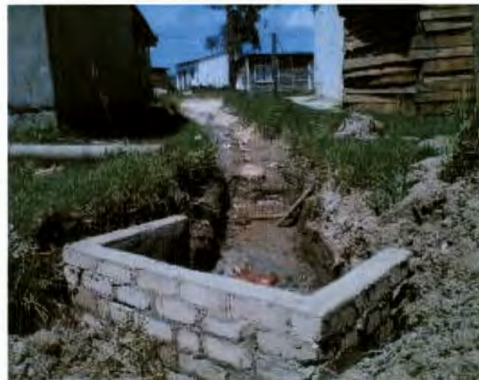
Storm water culvert and channel in response to the bad drainage of the site. (Benjamin, Social Impact Assessment .)
