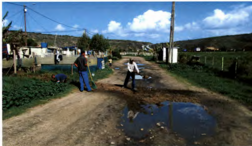
Pooling around the informal dwellings caused by bad drainage and a low water table
