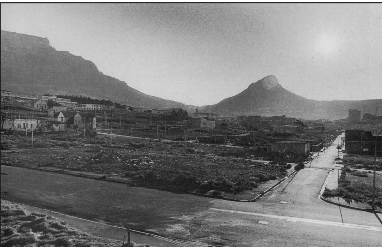
62 | Before and after demolition
